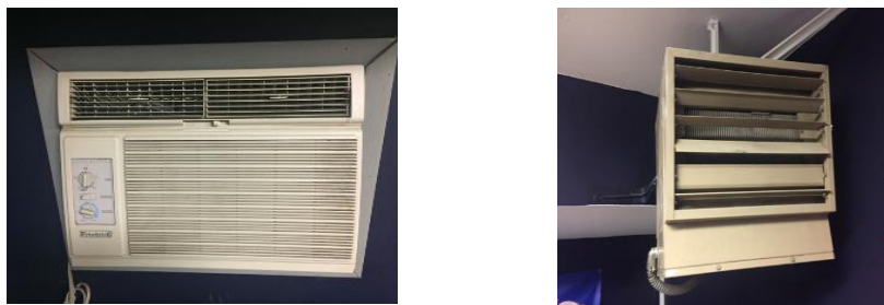
Image 3: Cooling & Heating System
