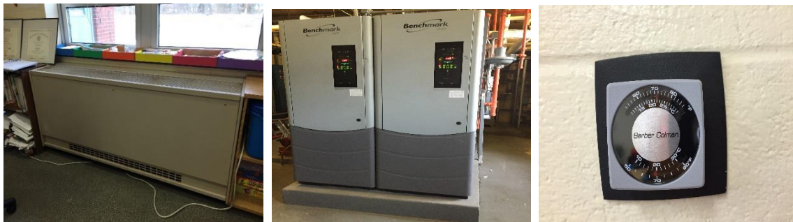
Image 3 Boiler, terminal unit and thermostat samples at the school
