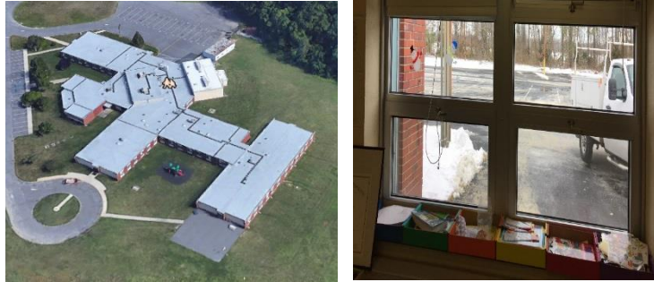
Image 1 Building roof and sample of windows
