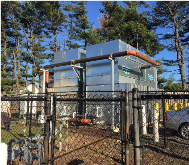
Image 15: Evapco Cooling Tower
