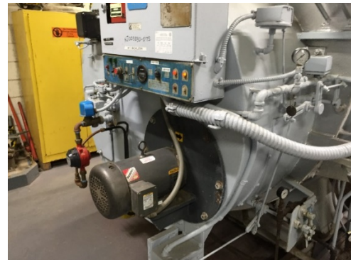
Image 10: 7 1/2 hp Boiler Blower Motor
