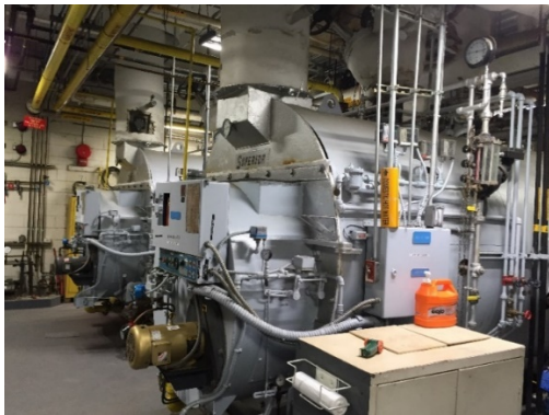
Image 9: (2) Superior Steam Boilers
