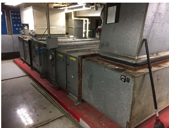
Image 7: AHU30 Located in M.E.R. 8
