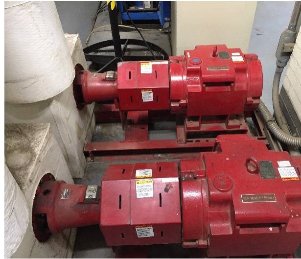
Image 16: (2) 25 hp Condenser Water Pumps
