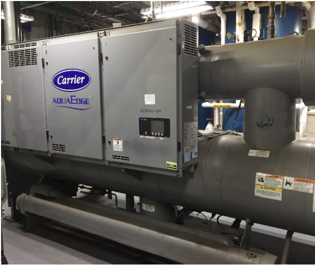
Image 13: New CH1 Located in Boiler Room
