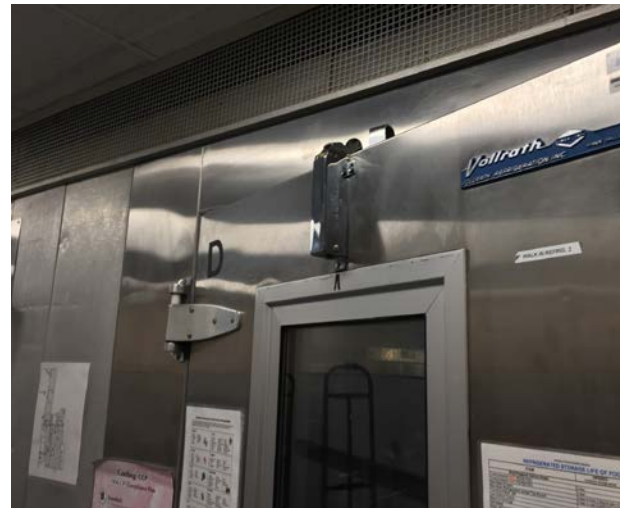
Image 24: Kitchen Equipment Walk-in Freezer
