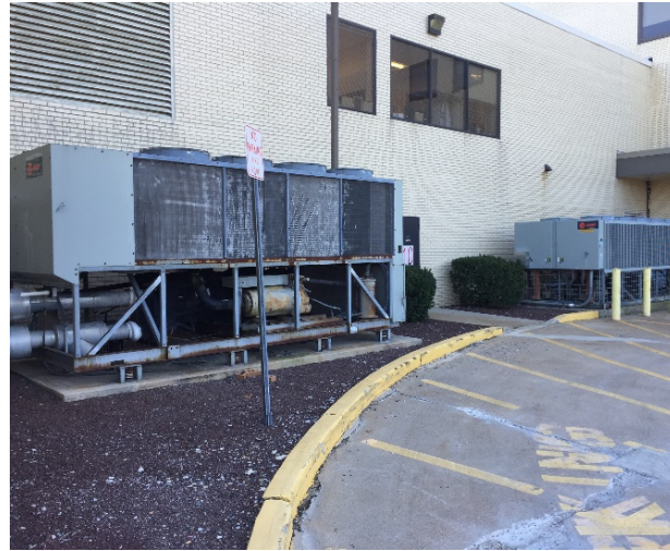
Image 14: Trane CH3 and CH4 Outside M.E.R. 8
