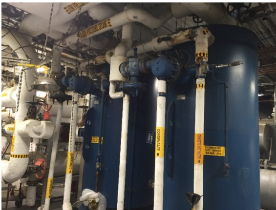
Image 19: DHW Storage Tanks
