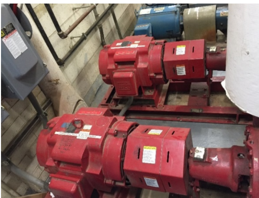
Image 11: (2) 25 hp Heating Hot Water Pumps
