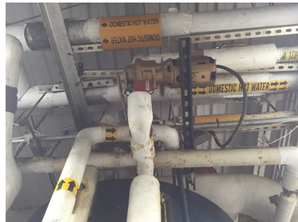
Image 20: DHW Supply Pumps
