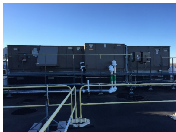
Image 8: AHU 39 Located on the Roof
