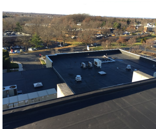
Image 2: Roof with EPDM Membrane
