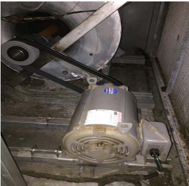
Image 8: Supply & Return Air Fan Motors
