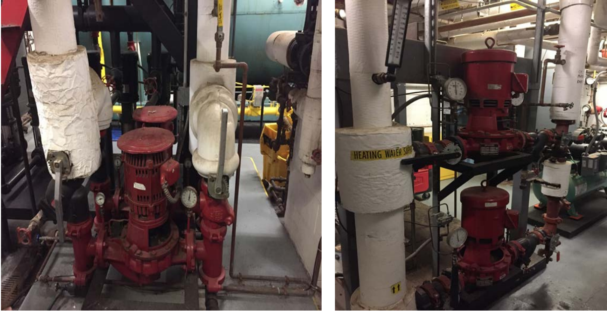
Image 15: Hot Water Pumps
