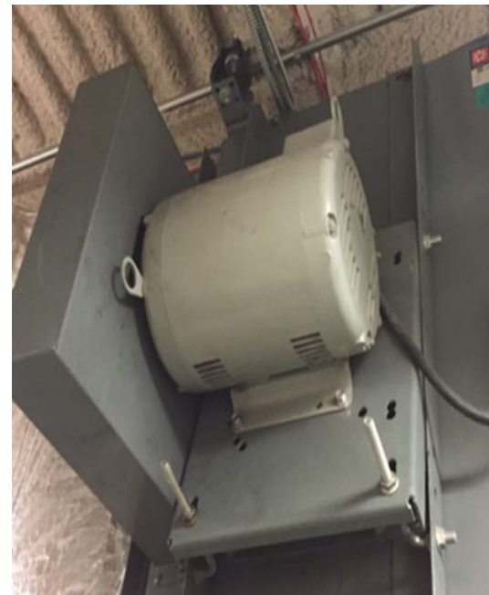
Image 8: Supply & Return Air Fan Motors
