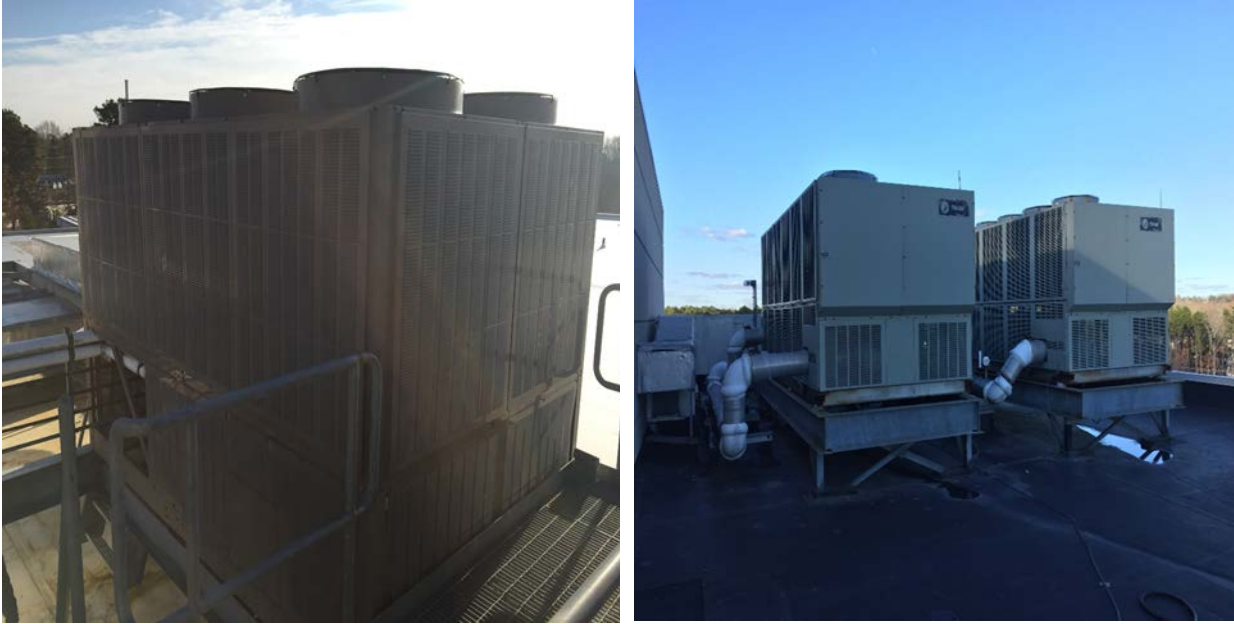
Image 24: York Air-Cooled Scroll & Trane Air-Cooled Screw Chillers
