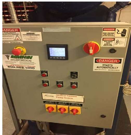
Image 28: Four Pumps Medical Vacuum System
