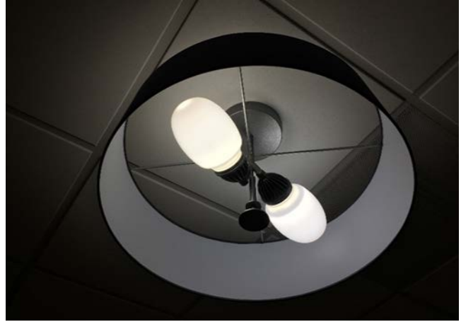
Image 6: Hallway Canopy (CFL) & Recessed LED Fixture
