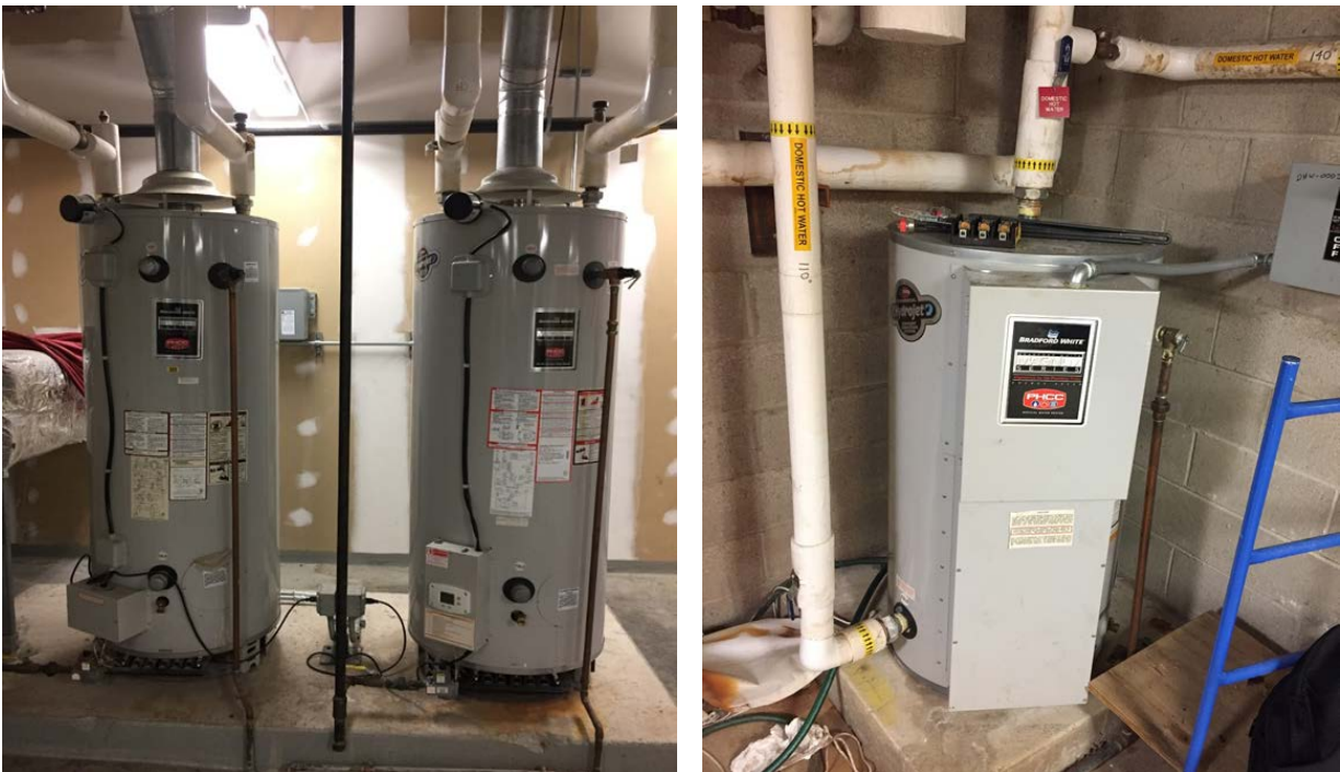
Image 32: Gas Fired & Typical Electric Water Heater
