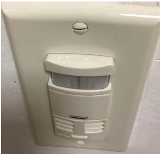
Image 8: Wall Mounted Occupancy Sensor & Timer
