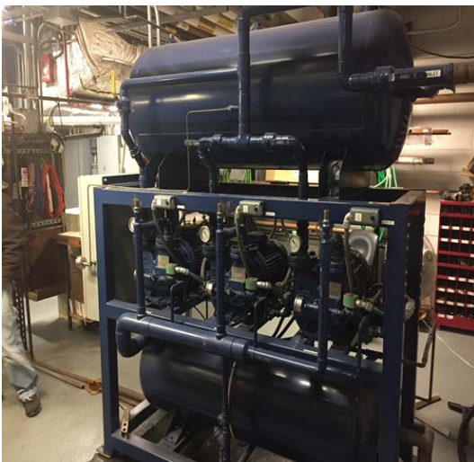
Image 28: Four Pumps Medical Vacuum System
