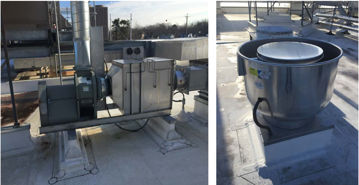
Image 11: Roof Mounted Exhaust Fans
