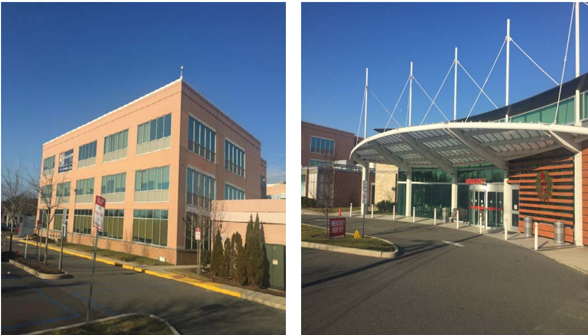
Image 3: Patient Tower & Emergency Area
