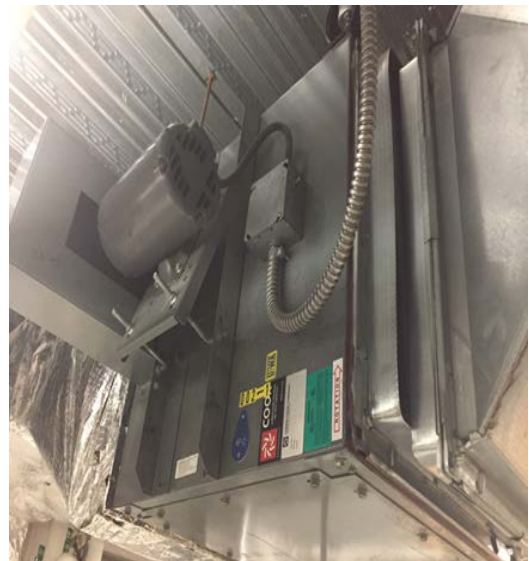
Image 6: Typical Constant Air Volume Unit with Return Air Fan Motor
