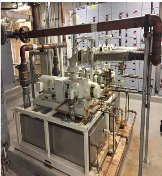
Image 29: Two Pumps Medical Vacuum System
