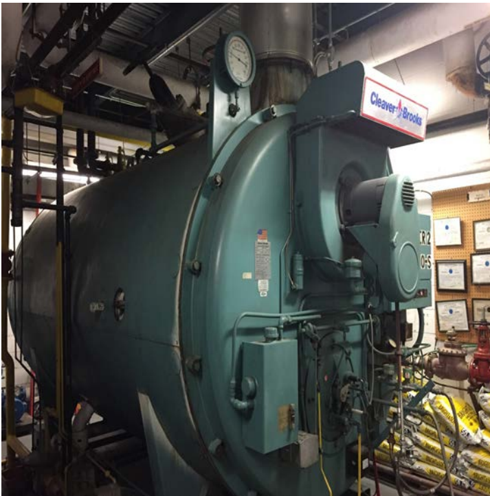
Image 12: Cleaver Brook Steam Boiler
