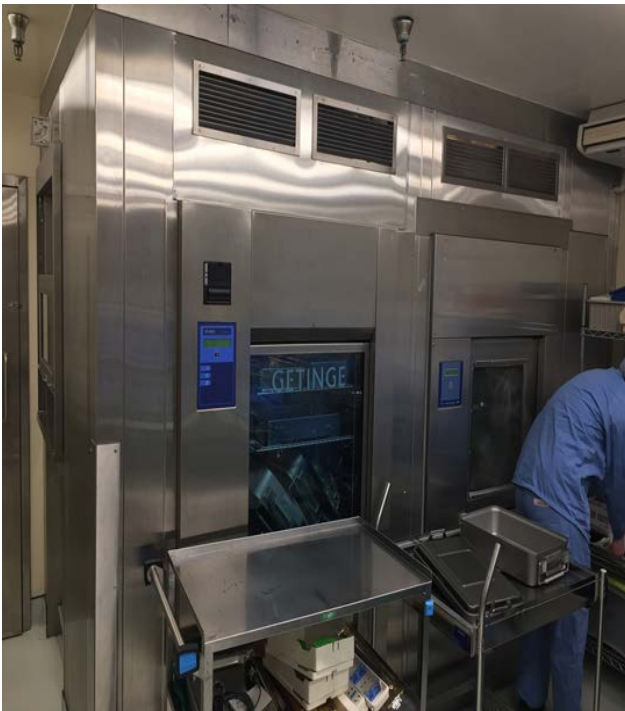
Image 14: Medical Steam Washer Disinfector & Humidifier
