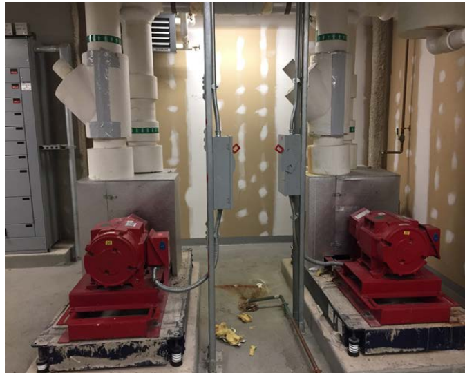
Image 27: 40 hp Chilled Water Pump
