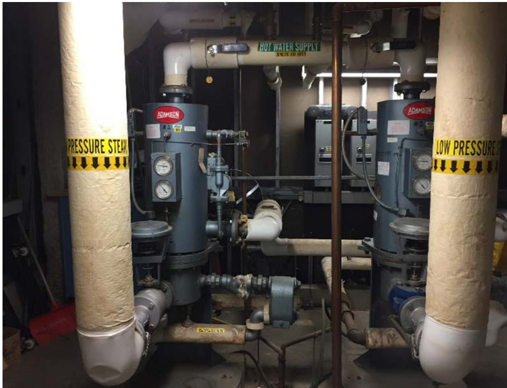
Image 31: DHW Through Low Pressure Heat Exchangers
