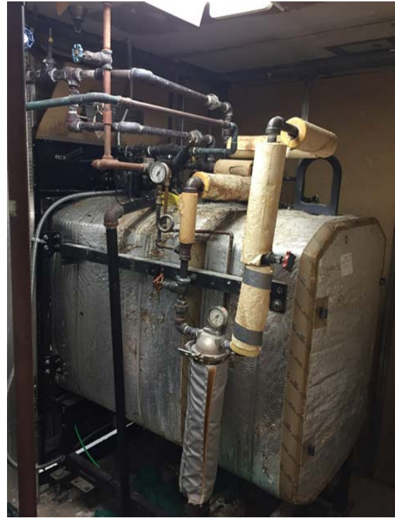
Image 13: Amsco 300 & 400 Series Sterilizers & Steam Jacketed Chamber
