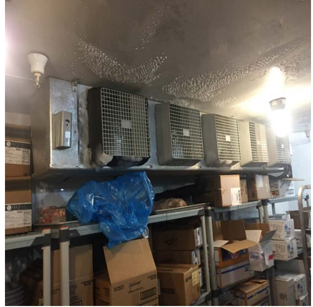
Image 19: Standup Solid Door Refrigerator & Walk-in Cooler
