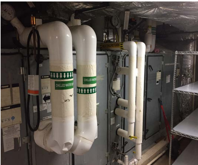
Image 6: Typical Constant Air Volume Unit with Return Air Fan Motor
