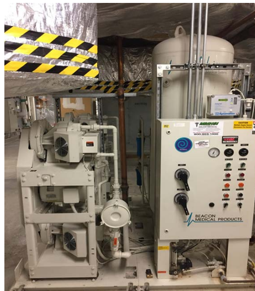
Image 29: Two Pumps Medical Vacuum System
