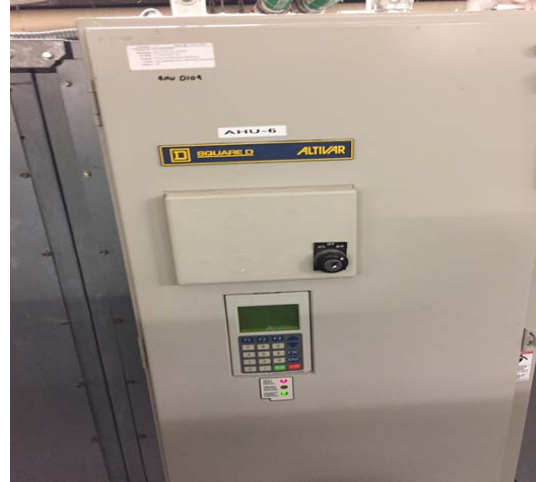
Image 7: Typical Variable Air Volume Unit with VFD Control
