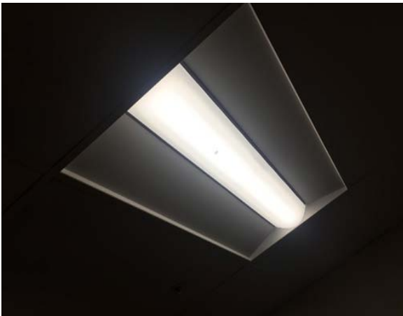
Image 4: Typical Recessed LED & T8 Fixtures
