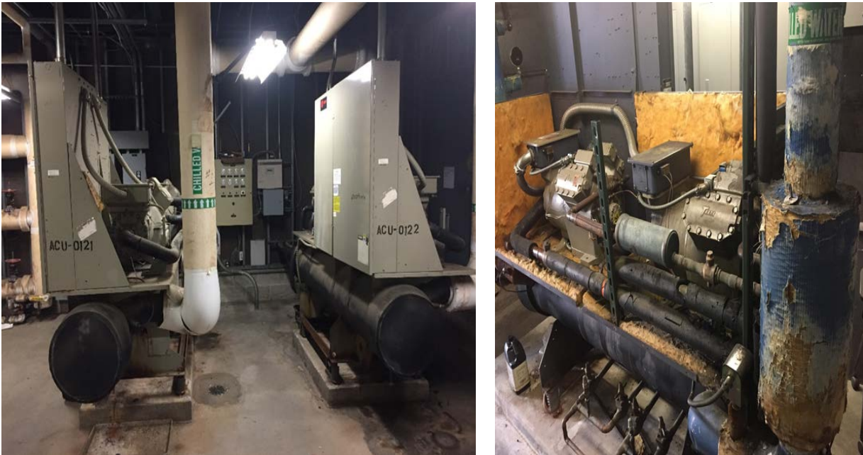
Image 25: Trane Reciprocating Chillers
