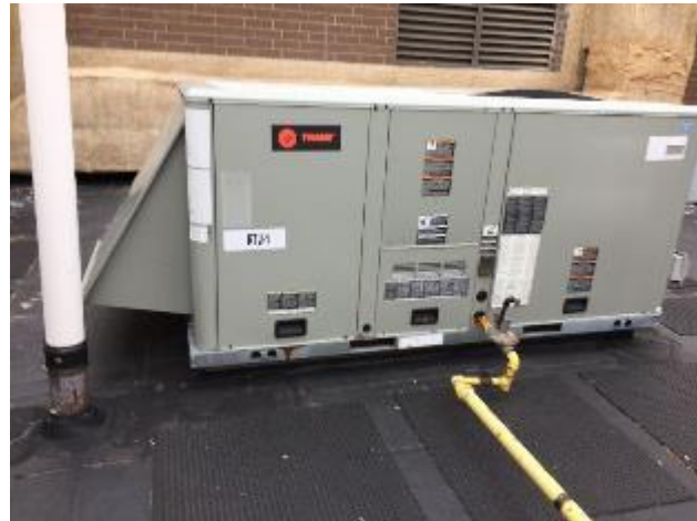
Image 9 Trane package AC w/gas heat
