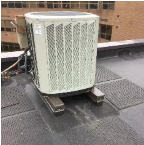
Image 8 Typical split-system AC condenser
