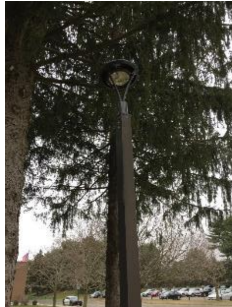
Image 3 Pole mounted LED fixture
