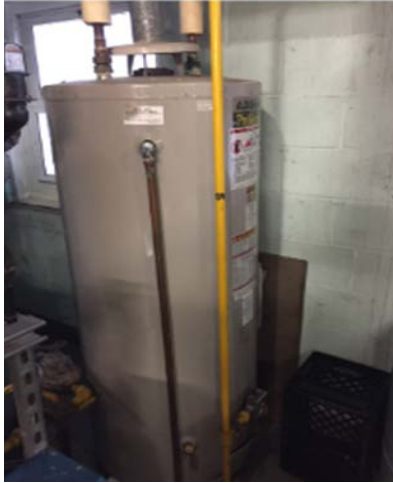
Domestic Hot Water Heater
