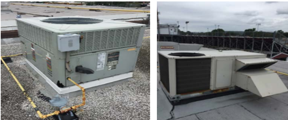
Roof Top Packaged Units
