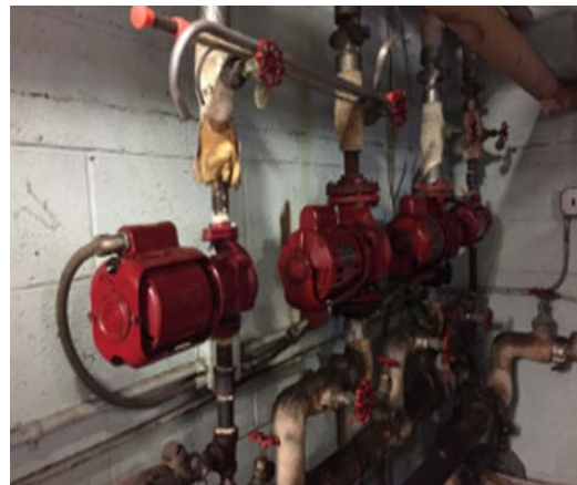
Four Heating Hot Water Pumps
