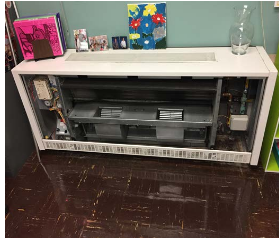
Typical Classroom Unit ventilator
