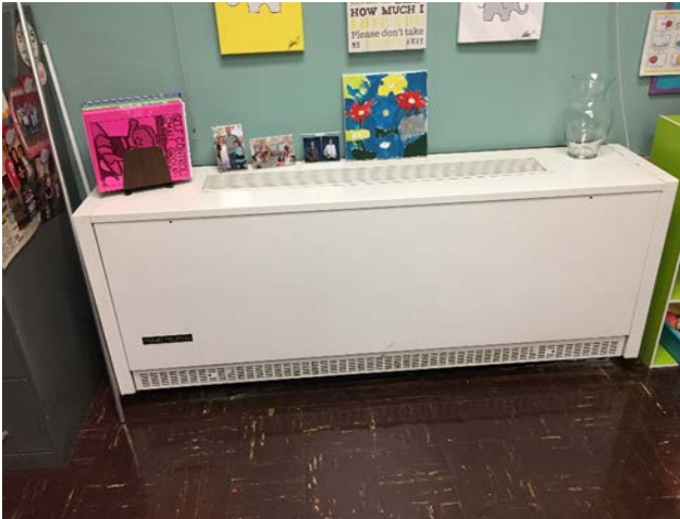
Typical Classroom Unit ventilator
