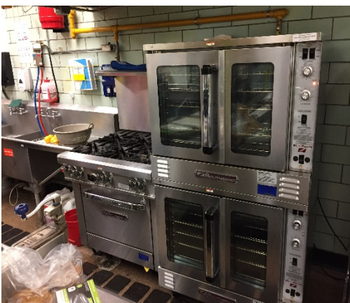
Convection oven and gas-fired cooking range
