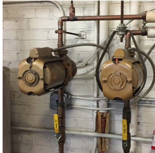
DHW & Circulating Pumps
