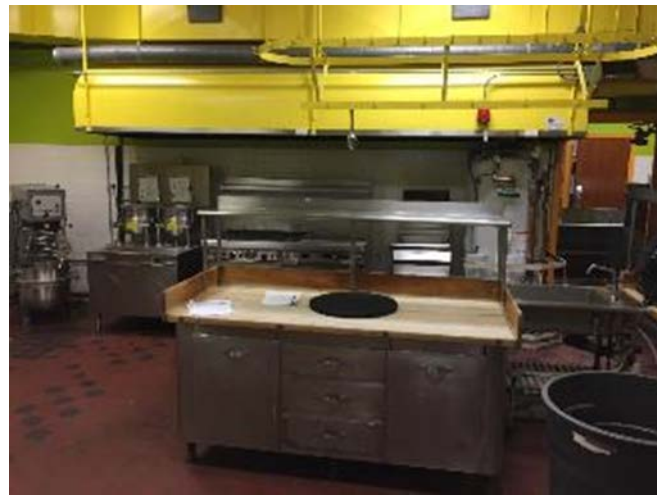
Other Kitchen Equipment
