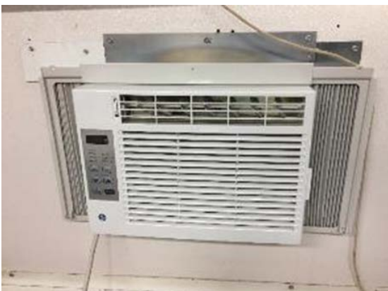
Direct Expansion Cooling System
