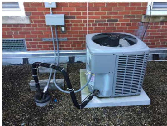
Direct Expansion Cooling System
