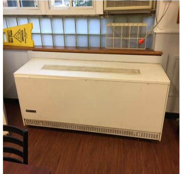
Steam Boiler & Unit Ventilator
