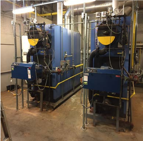
Steam Boiler & Unit Ventilator
