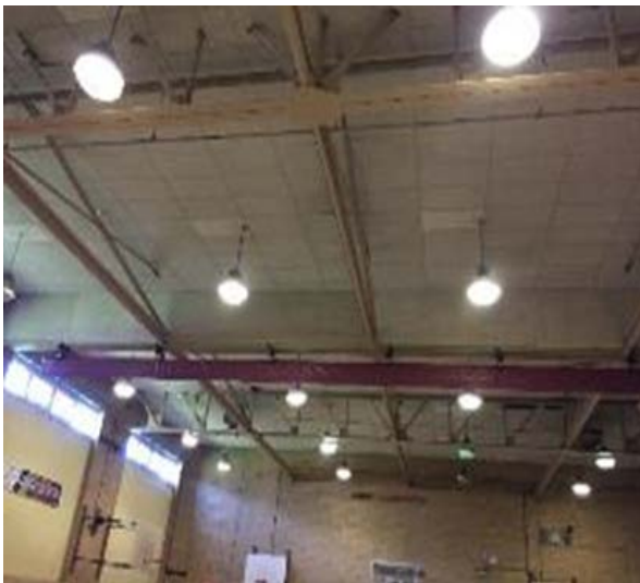
Gym Metal Halide & LED Exit Sign
