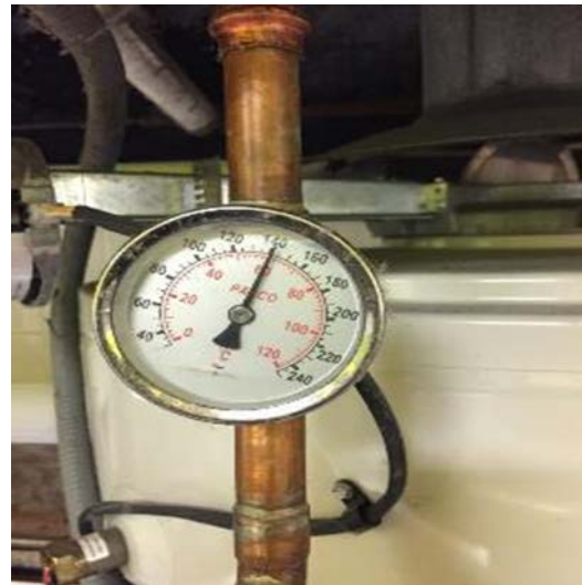
Storage Tank Water Temperature Indicator
