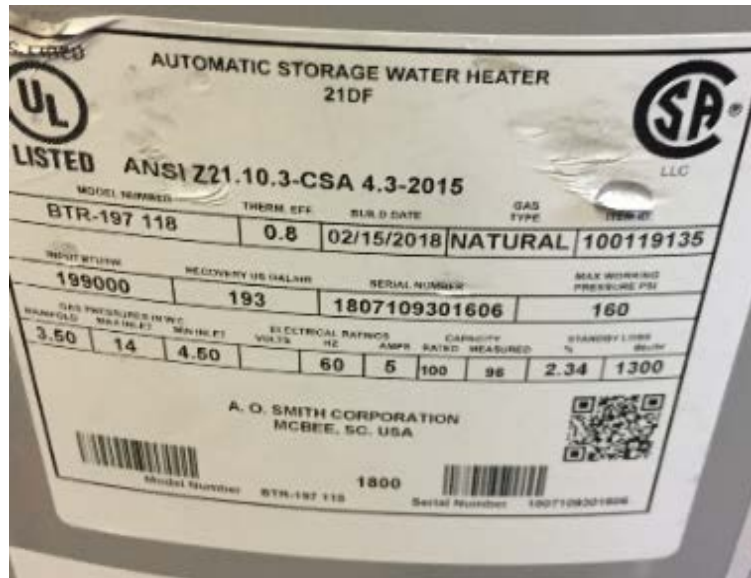
Hot water Heater Nameplate
