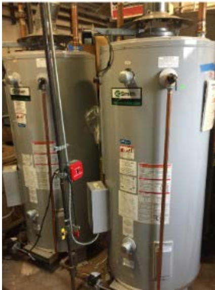
Hot water Heater
