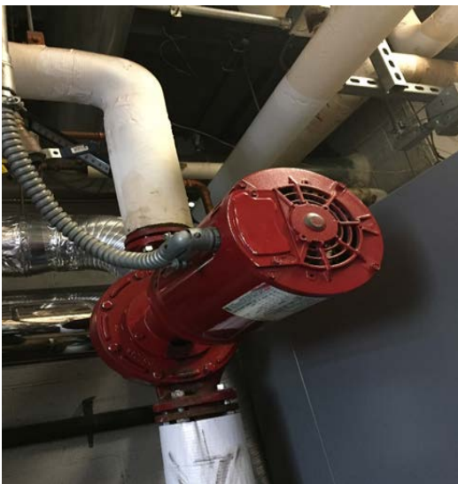
2 hp Hot Water Pump and Unit Ventilator
