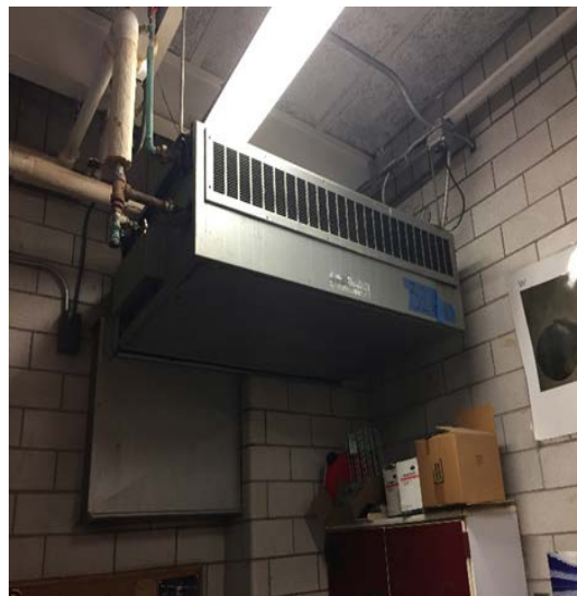
2 hp Hot Water Pump and Unit Ventilator
