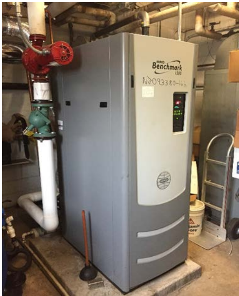
Aerco Hot Water Boiler and Its Control Scheme
