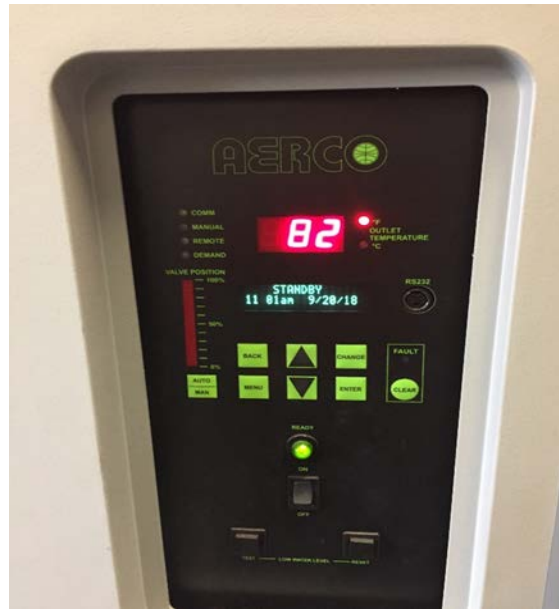
Aerco Hot Water Boiler and Its Control Scheme
