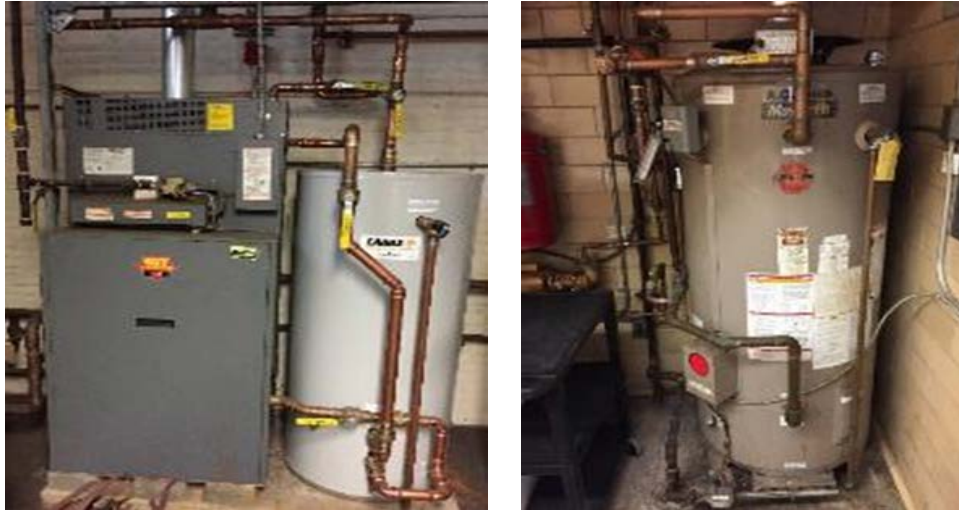
Domestic Hot Water System
