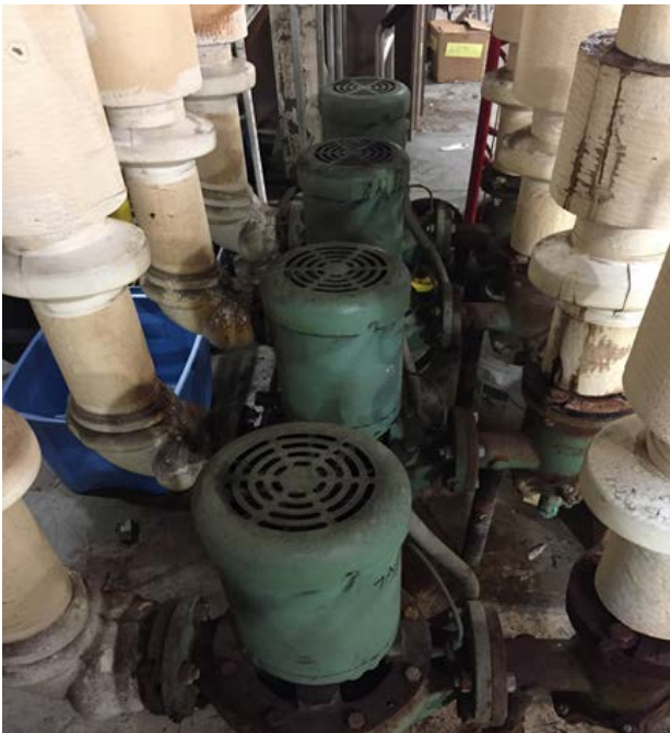
Hot Water Heating System
