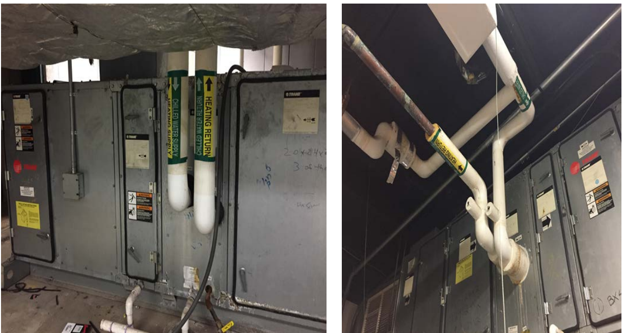
AHUs with Chilled & Hot Water Coils
