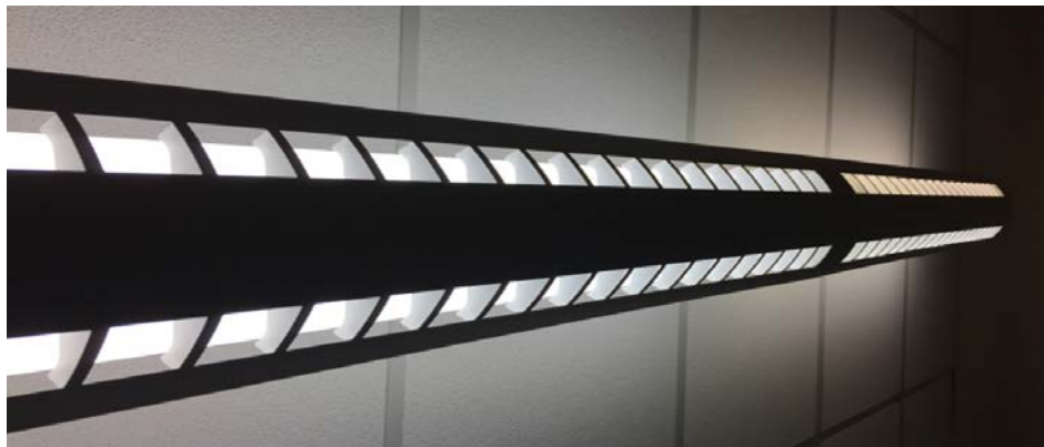
Typical Interior Lights & Occupancy Sensors
