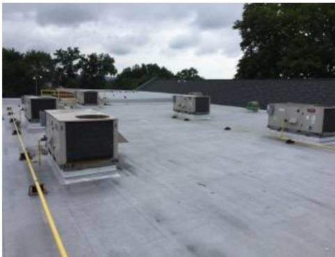
Package ACs on roof
