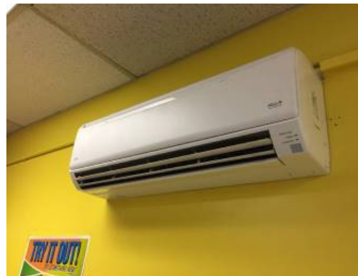
Split AC (Cafeteria)
