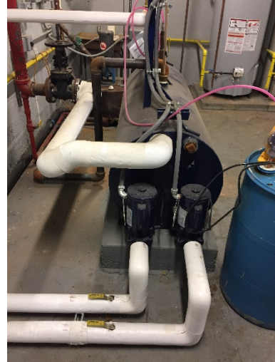
Condensate Tank and Feed Pumps
