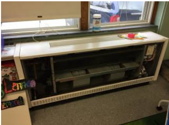
Unit Ventilator in classroom
