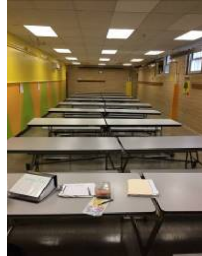
Cafeteria T8 Fixtures
