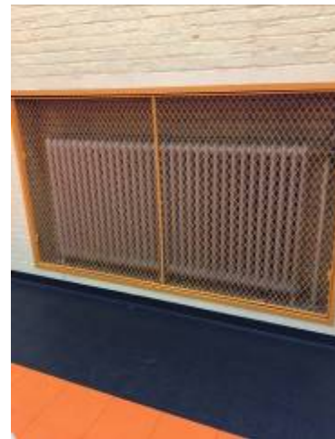
Radiators in Gym
