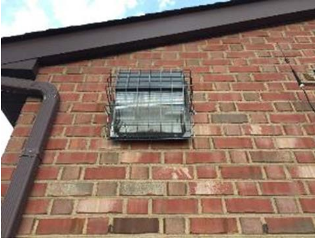
Exterior Wall Pack Fixtures
