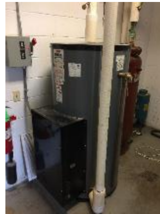
Electric water heater serving the C-wing
