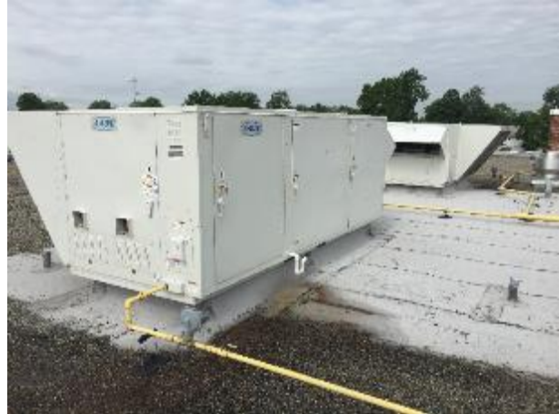
Roof top unit
