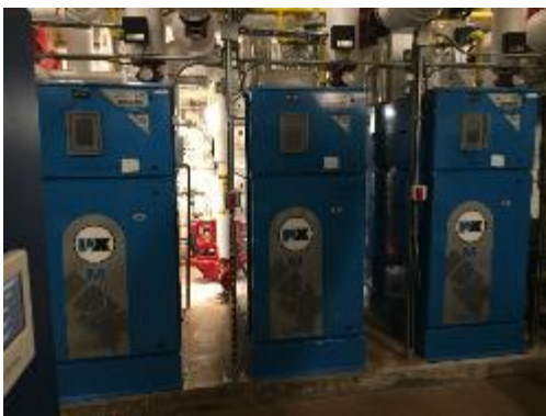
Mach C-3000 boilers
