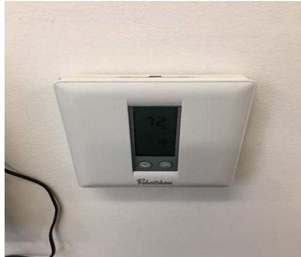
Programmable Thermostat
