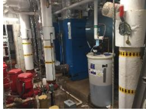
Hot water pumps
