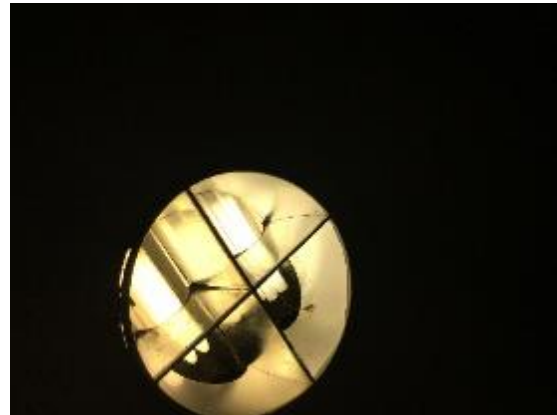
Recessed CFL fixtures
