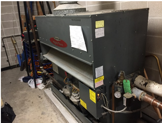
Water heater serving the locker rooms (needs replacement)
