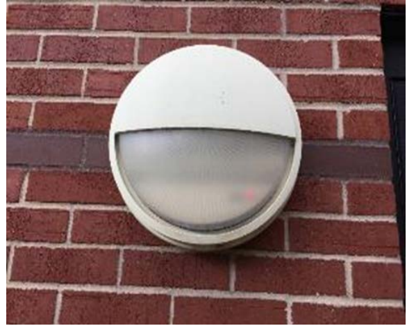
Exterior Wall Pack Fixtures
