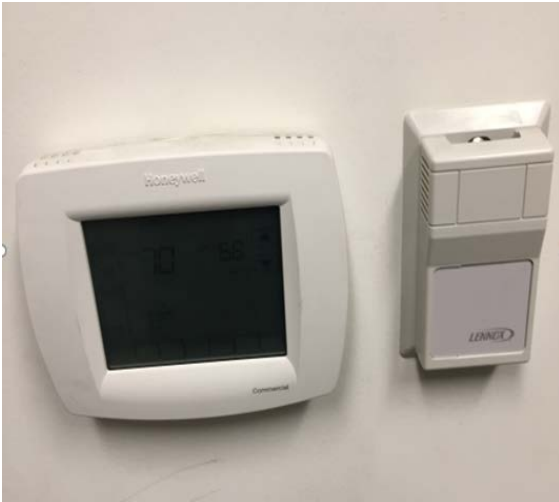
Programmable Thermostat
