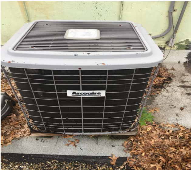
Direct Expansion Cooling System
