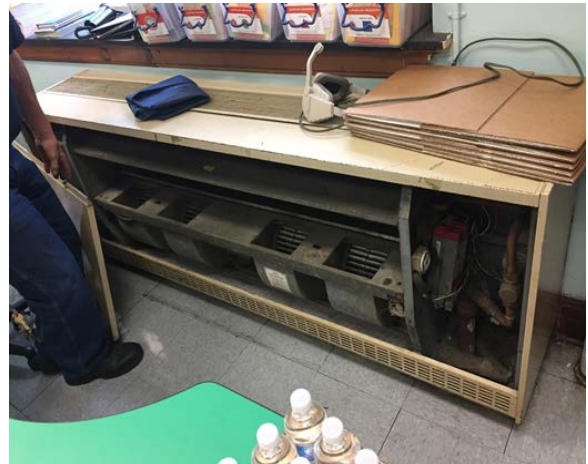
Typical Classroom Unit Ventilator
