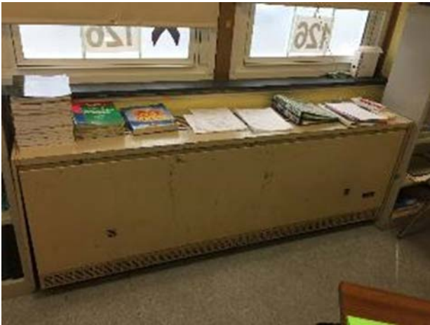
Typical Classroom Unit Ventilator
