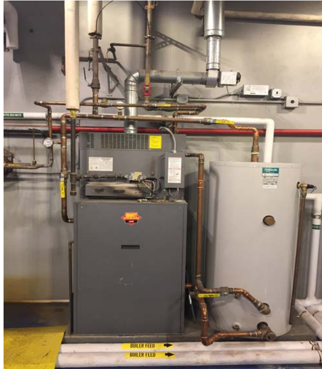
Domestic Hot Water Heater
