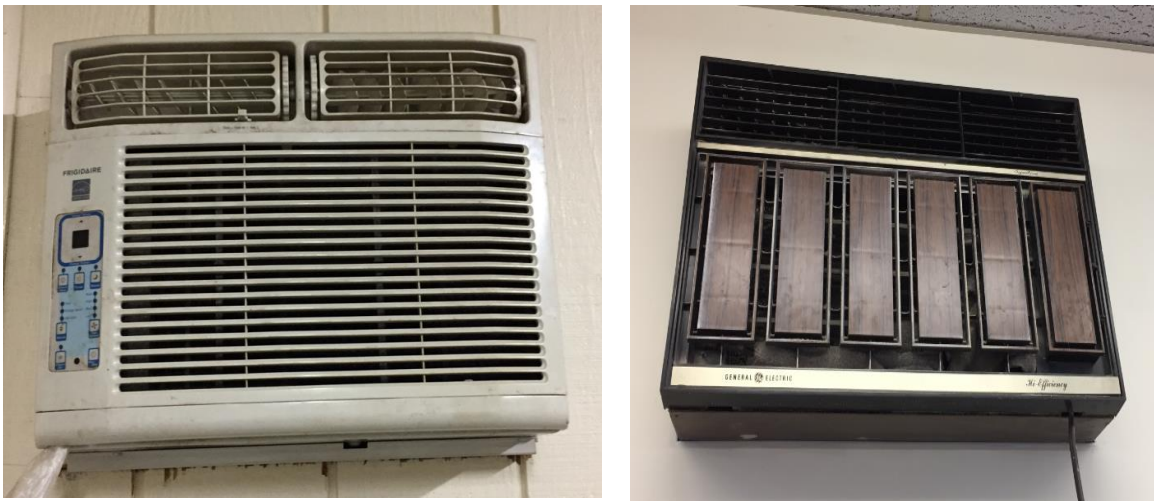
Image 14: Window AC Units
