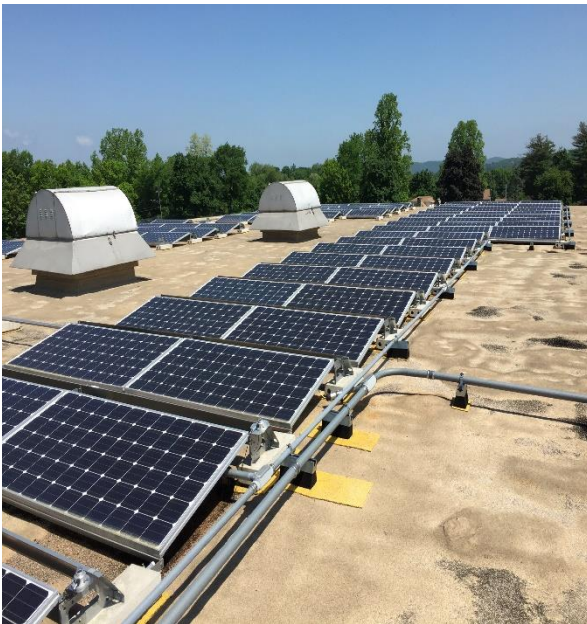
Image 5: Roofing Membrane with PV Arrays
