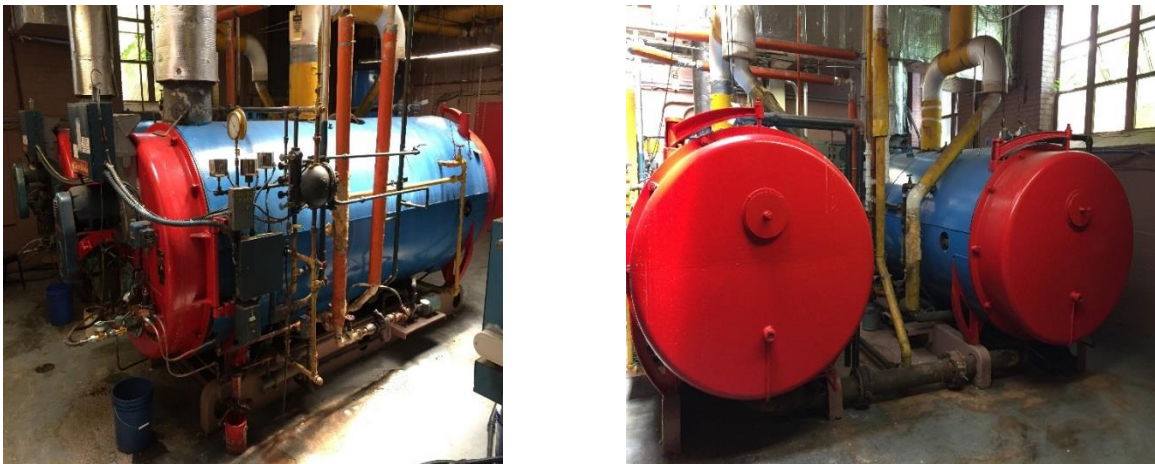
Image 9: Cleaver Brook Steam Boilers
