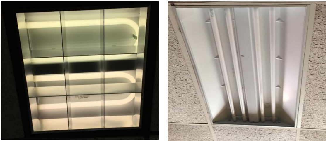
Image 7: Typical Interior Lighting System
