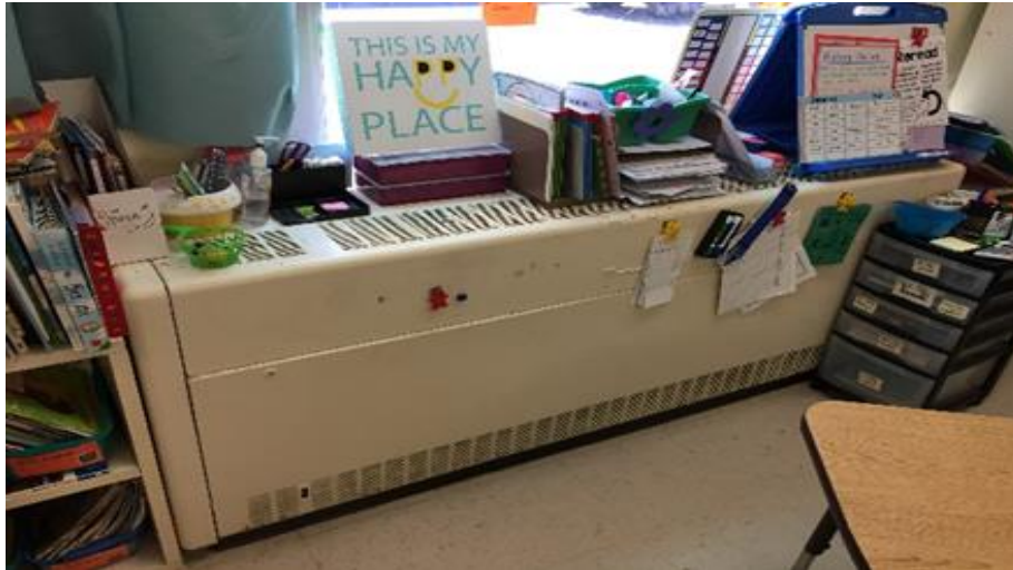
Image 10: Classroom Nesbitt Unit Ventilator
