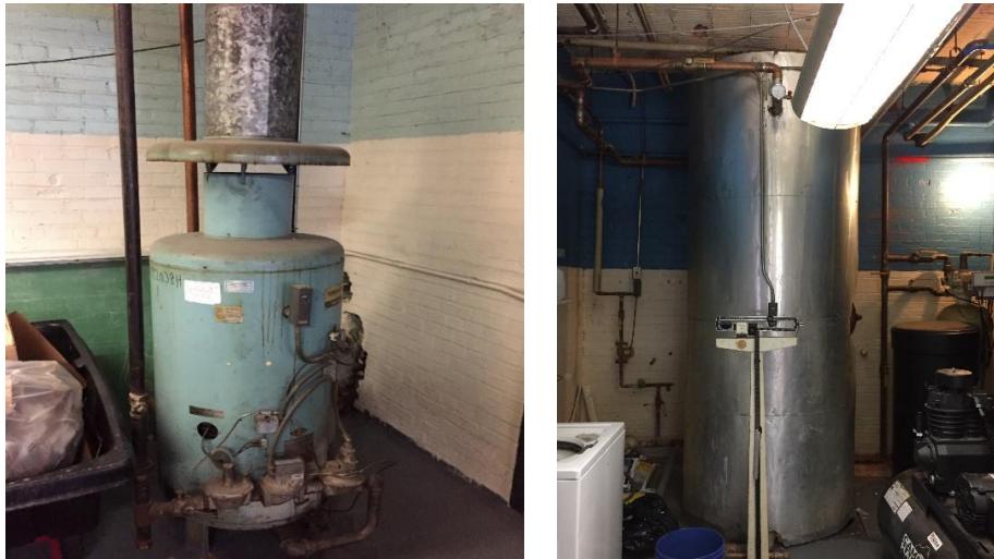
Image 16: Domestic Water Heating System
