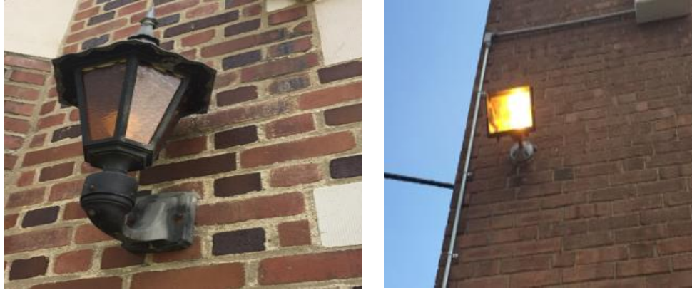
Image 8: Exterior Wall Packs
