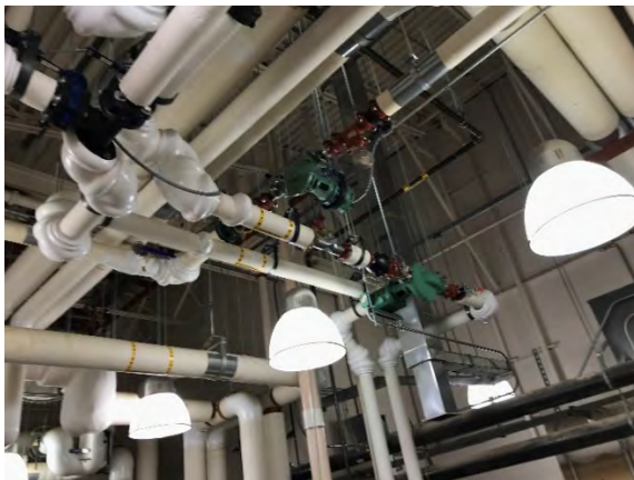
Heating Hot water pumps
