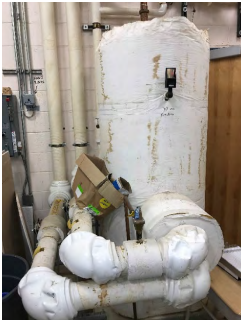
DHW Storage Tank
