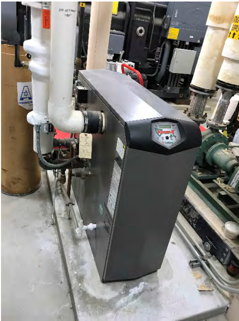
Indirect Hot Water System
