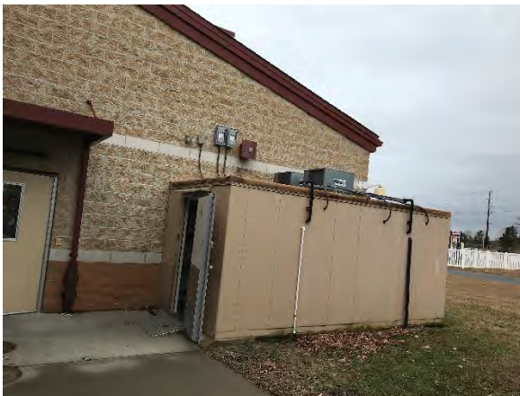
Exterior Walk-in Units
