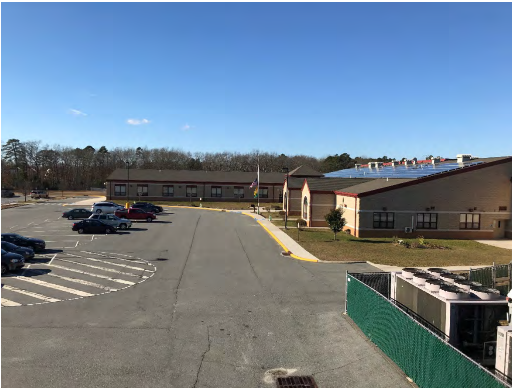
Solar Panels on Roof
