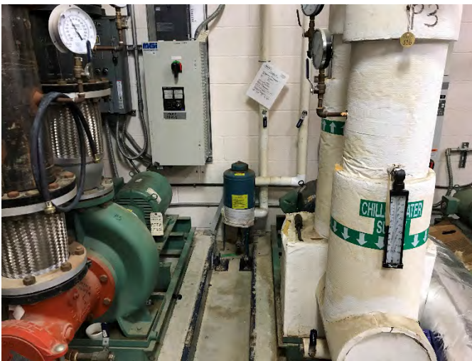
Chilled Water Pumps
