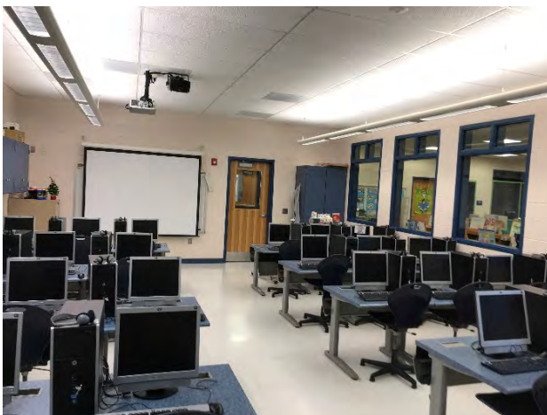
Computer Room Lighting
