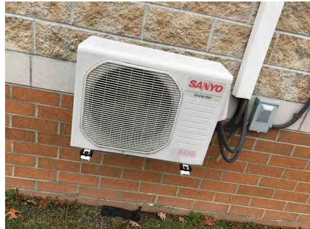
Outdoor Condensing Unit
