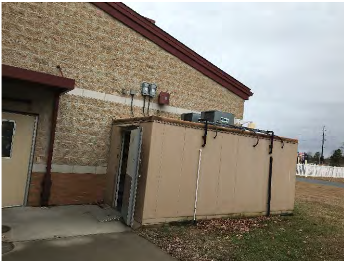
Walk in Freezer and Cooler
