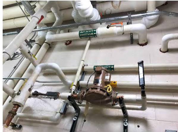
DHW supply Pump
