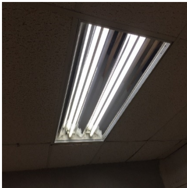
4-foot T8 linear fixtures
