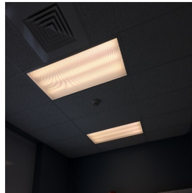
4-foot T8 linear fixtures
