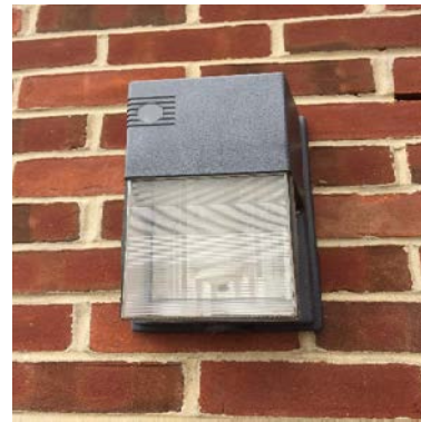
Compact fluorescent lamp fixtures
