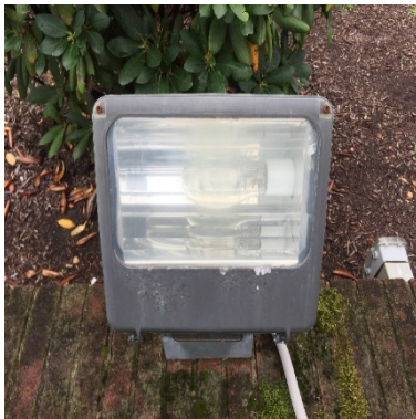
High pressure sodium fixtures
