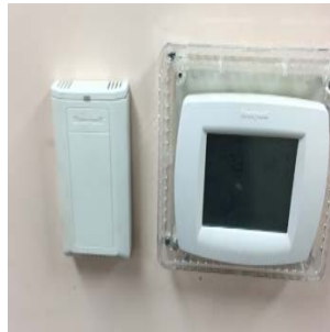
Indoor Thermostat Control
