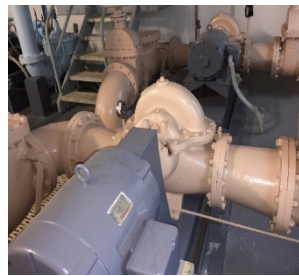
DPW plant 2 High Service Pumps
