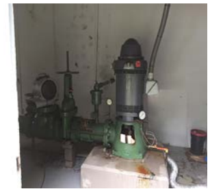
Well 11 - 125 hp pump
