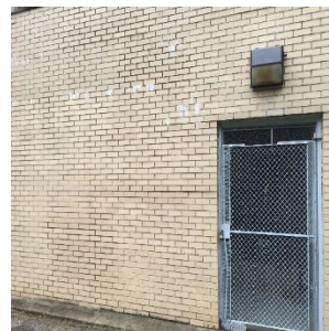
Exterior Metal Halide lamp fixture
