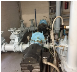
DPW plant 2 Backwash Pumps
