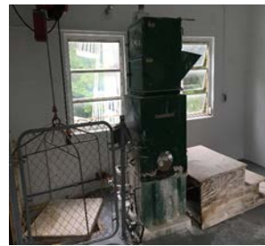
DPW plant 2 Water Treatment Equipment
