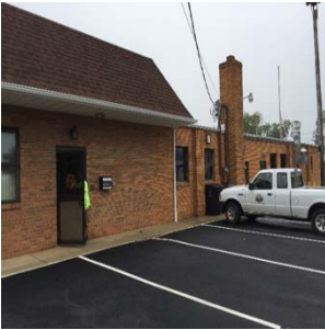
Building Walls & Roof
