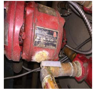
Hot water Pump nameplate
