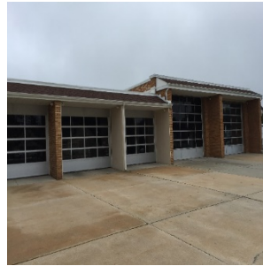
Exterior Rolling Doors
