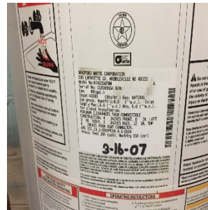
DHW Heater nameplate
