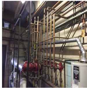
Hot water piping system
