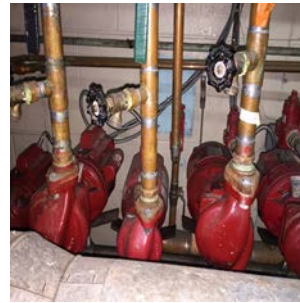
Hot water pumps
