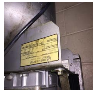
Air compressor nameplate
