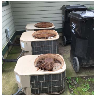
Outdoor Condensing Unit
