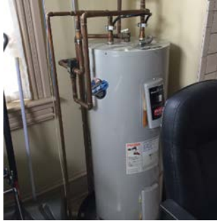
Domestic Hot Water Heater
