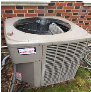
Outdoor Condensing Unit
