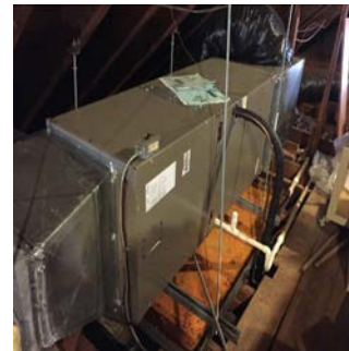
Air Handling Unit in the Attic
