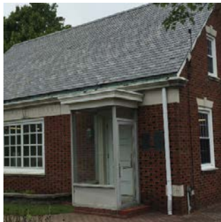
Main Library Exterior
