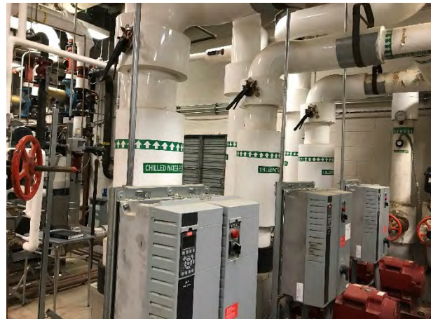
VFD Driven CHW Pumps
