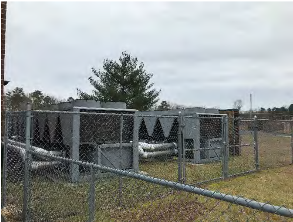
Chiller Plant Outdoor
