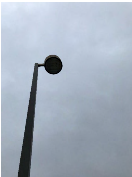
Pole Mounted Fixture
