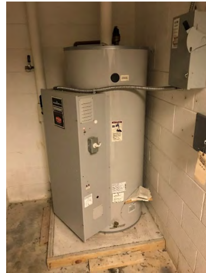
Electric Storage Tank Water Heater
