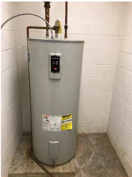
Electric DHW Heater
