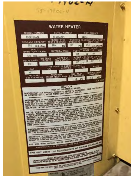
DHW Heater Nameplate
