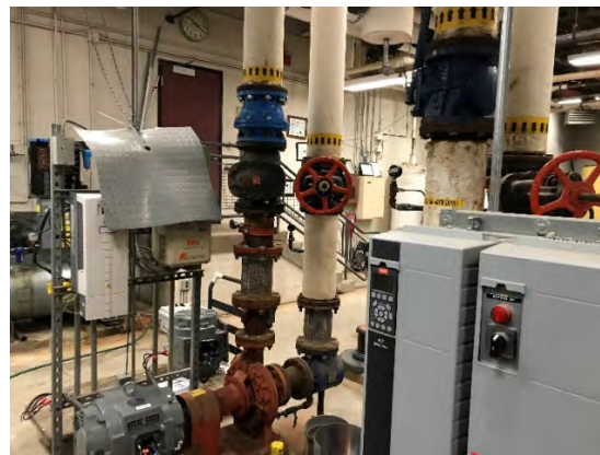
Heating Hot water pumps
