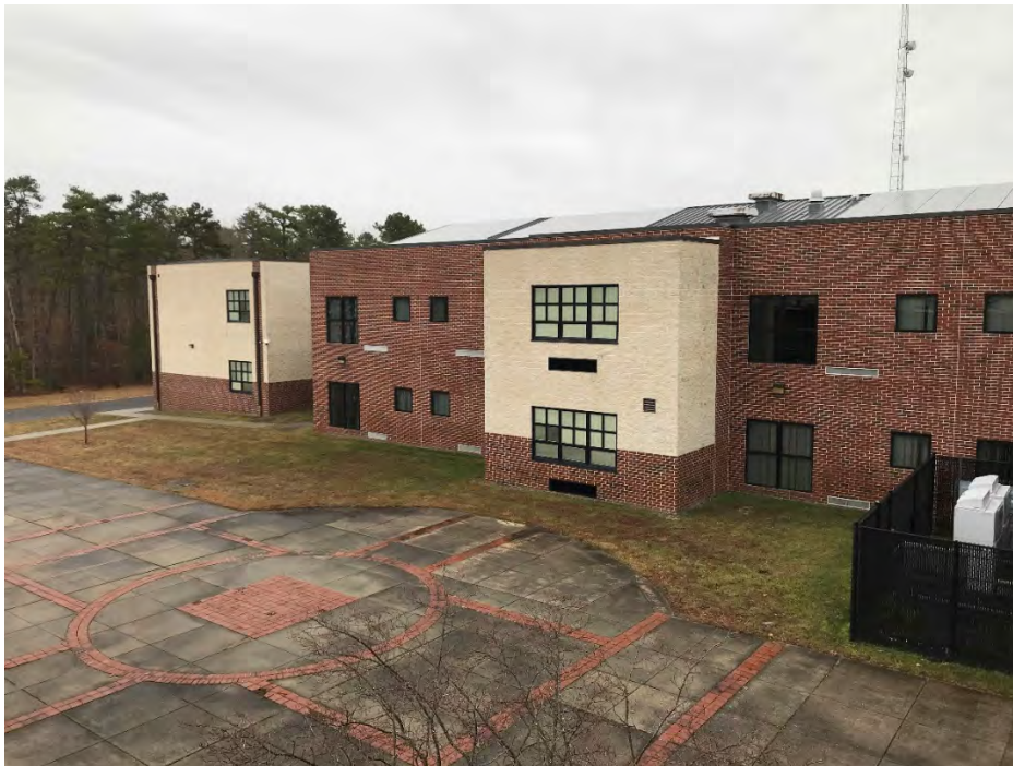
Solar Panels on Roof
