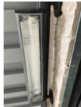
Door mounted fixture
