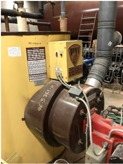
Natural Gas Storage Water Heater
