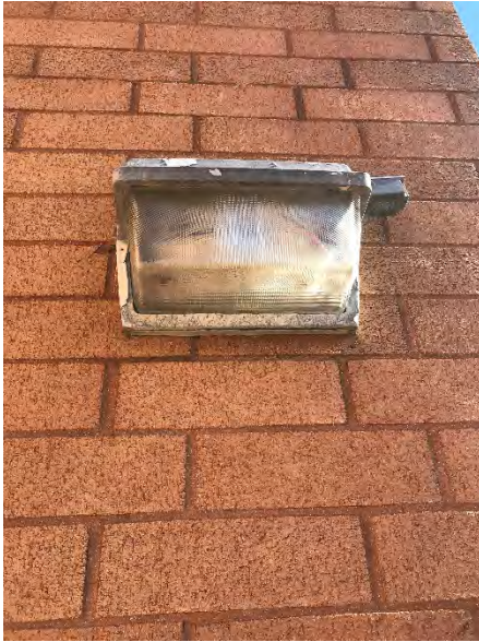
Wall Mounted Exterior Fixture
