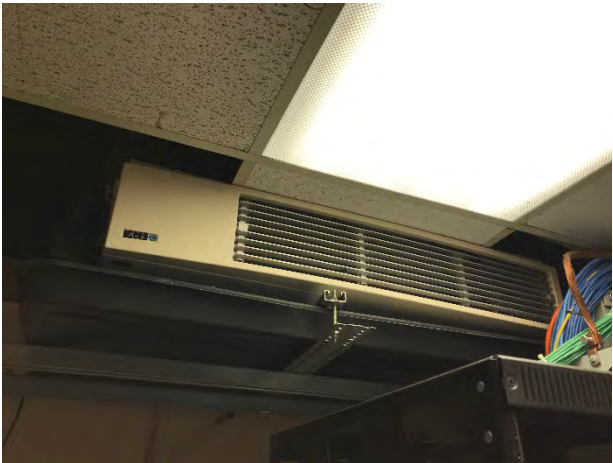
Split System Unit in IDF room
