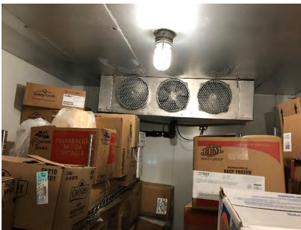
Freezer Evaporator fans
