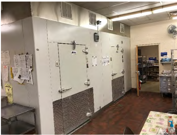
Walk In cooler and Freezer
