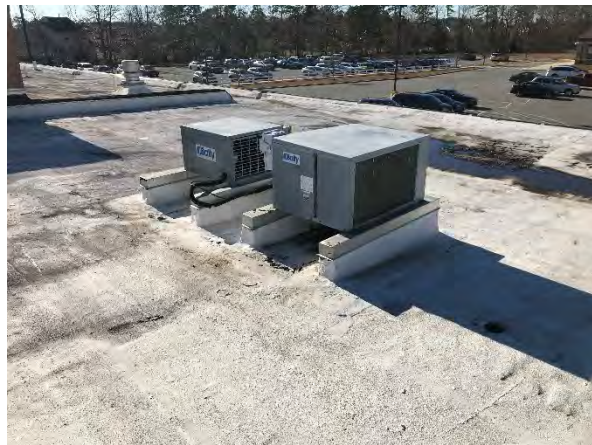
Compressor Units on Roof
