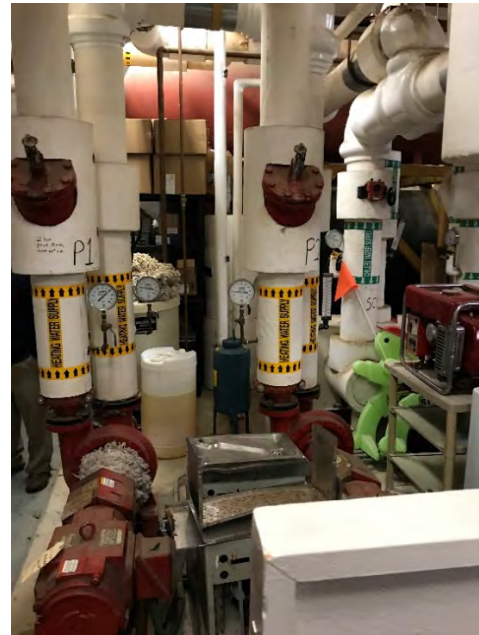
Heating HW Pumps
