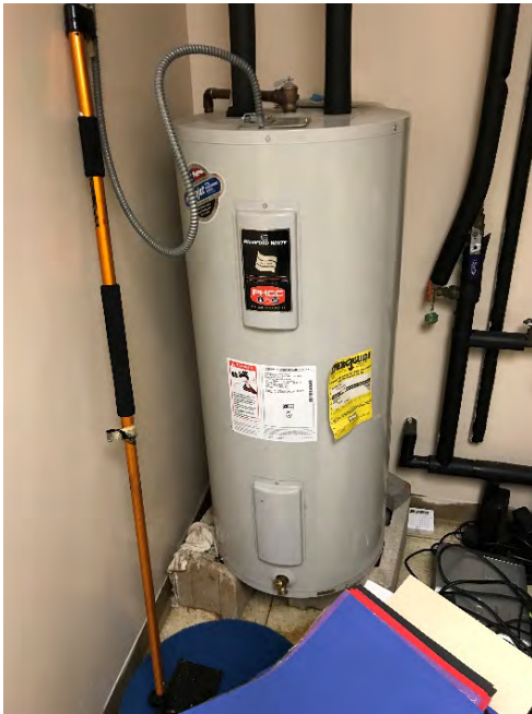
Electric DHW Heater
