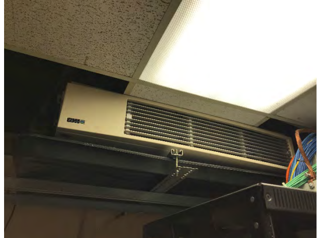
Server room lighting
