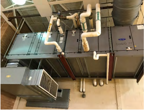
AHU in Gym
