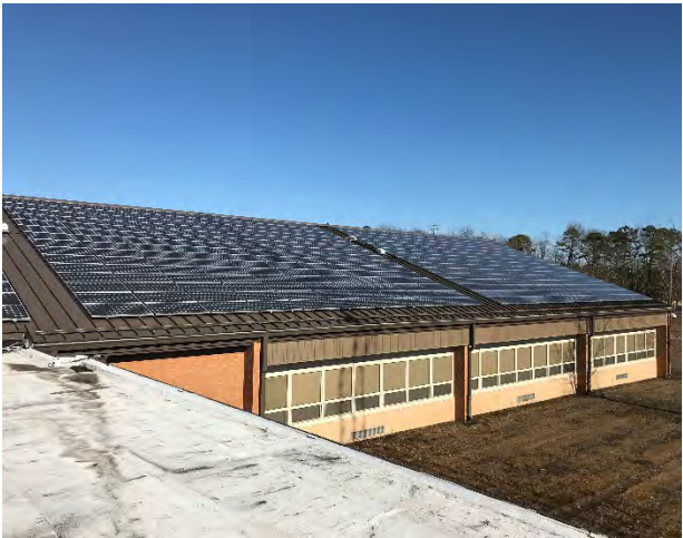
Solar Panels on Roof
