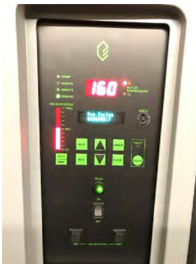
Boiler Front Panel
