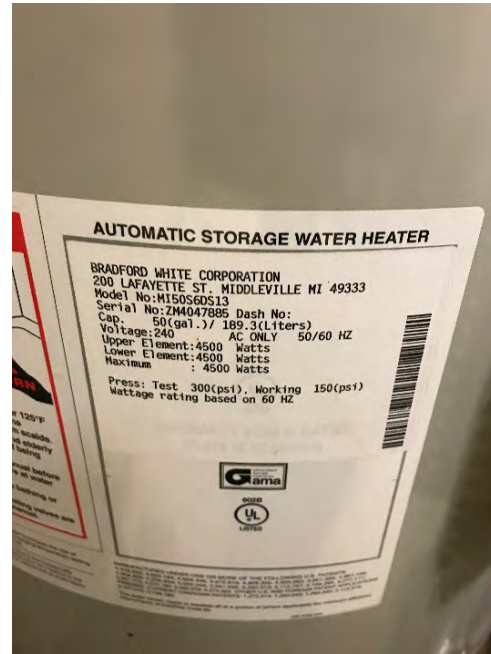
Electric DHW heater nameplate
