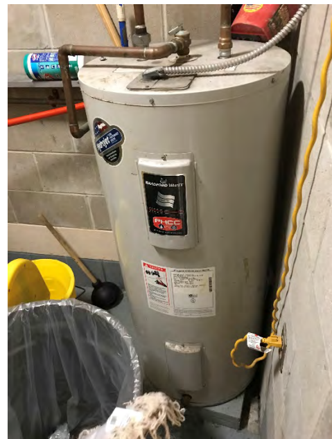
Electric Water Heater
