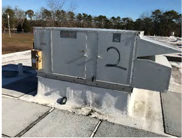
RTU on Roof
