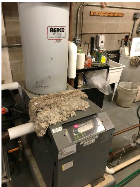
Gas fired DHW Heater
