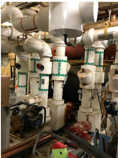
Chilled Water Pumps
