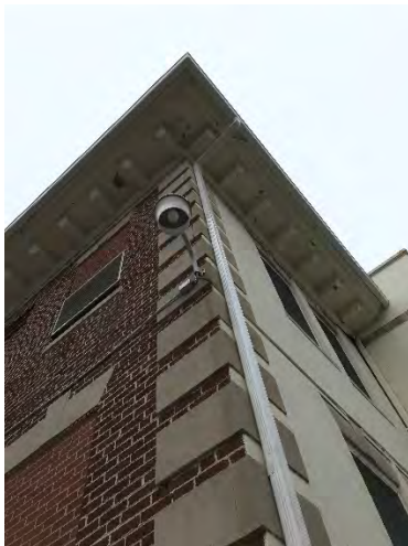
Exterior HID fixture
