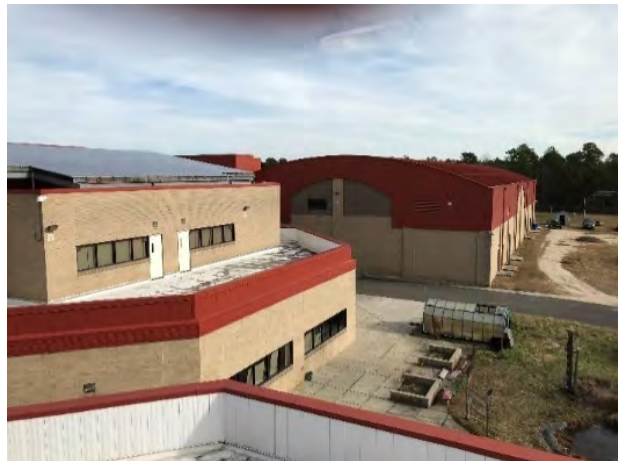
Lighting Fixture on Lower Roof
