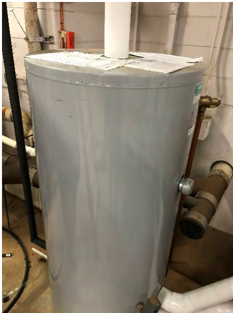
DHW Storage Tank
