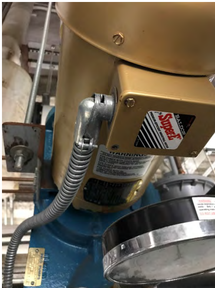
Heating Hot Water Pump
