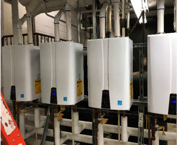
Hot Water Heaters
