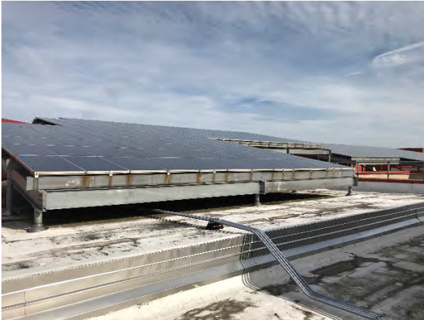
Solar Panels on Roof
