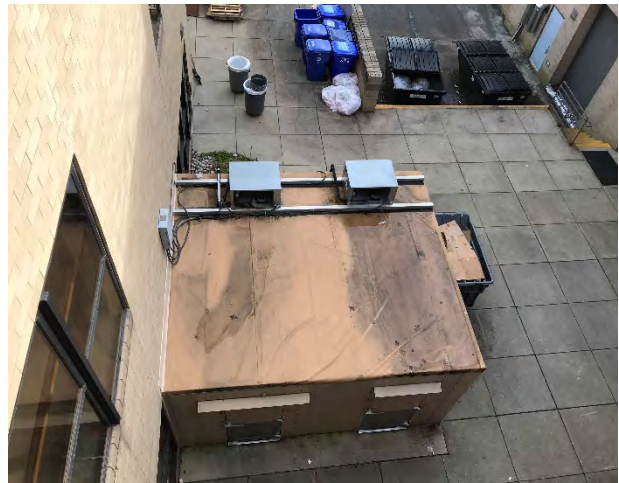
Walk in Cooler and Freezer
