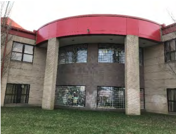
Canopy Mounted Lighting
