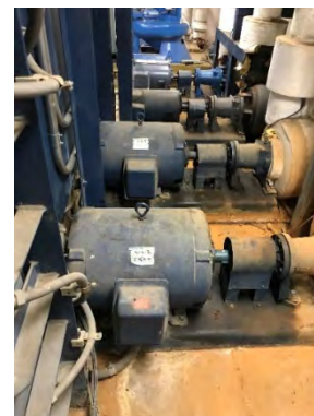
Chilled Water and Condenser Water Pumps
