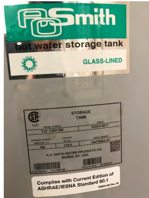
Storage Tank Nameplate
