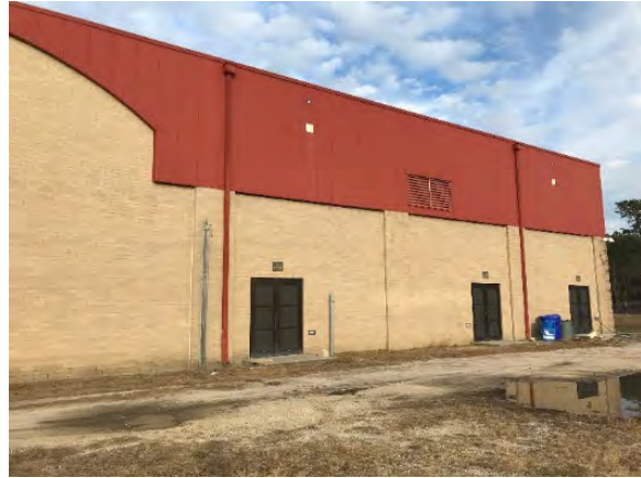
Wall Flush Lights on the Door
