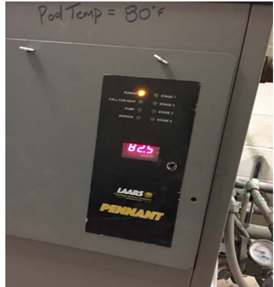
: Indoor Pool Heating Hot Water Boiler
