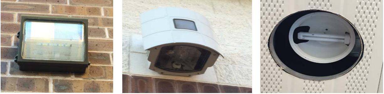
Image 1: Exterior Wall Pack & Recessed Fixtures
