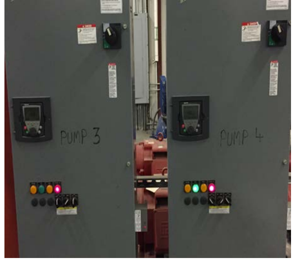
Hot Water Pumps & VFD Control System
