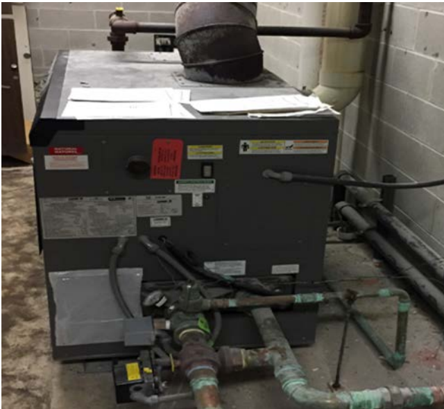
: Indoor Pool Heating Hot Water Boiler
