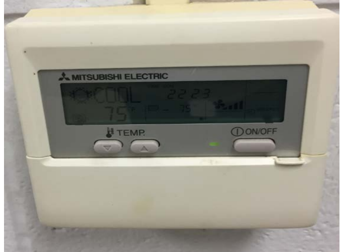
VFD Control & Programmable Thermostat
