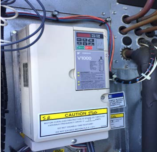
VFD Control & Programmable Thermostat
