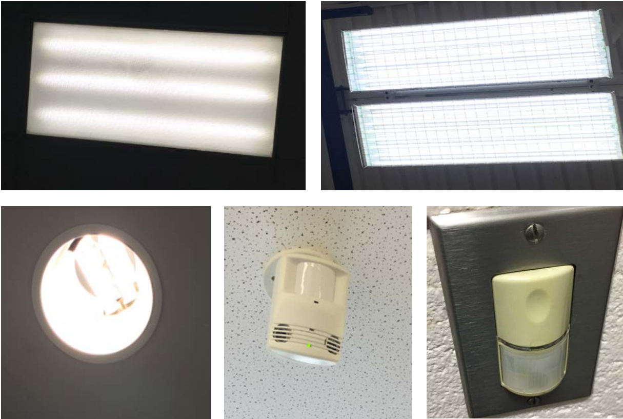
Interior Lighting & Occupancy Sensors
