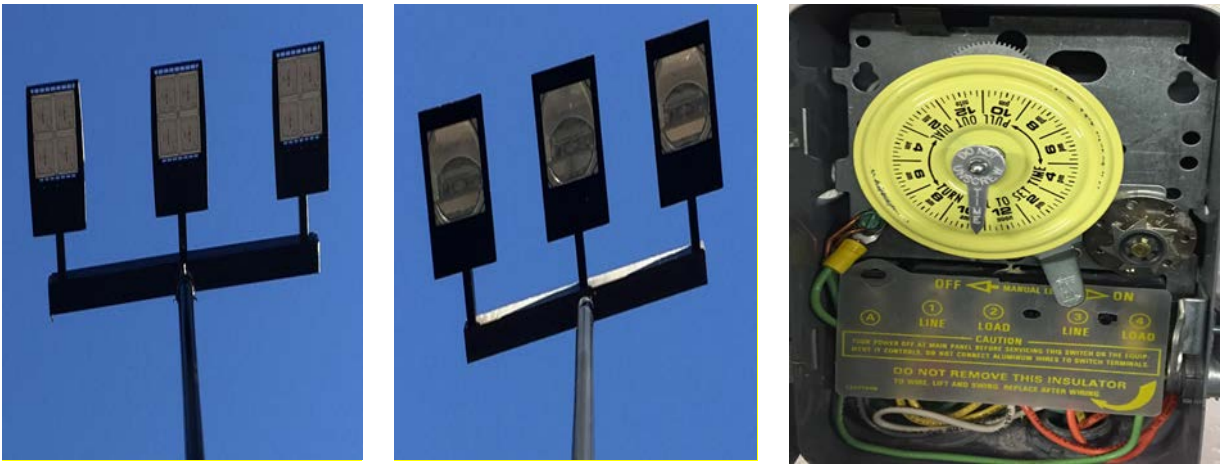
Image 2: LED, Metal Halide Pole Lights & Timer
