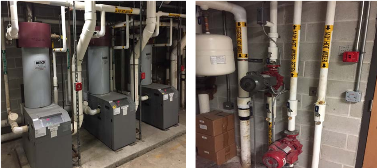
Domestic Hot Water Heaters
