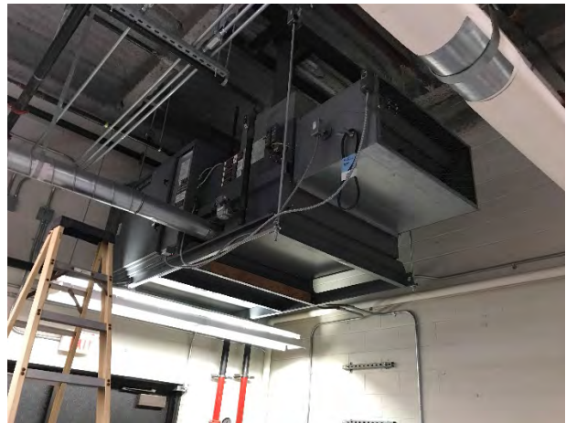
Make up air Unit in Boiler Room
