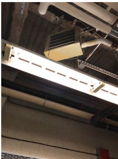
Boiler Room Lighting
