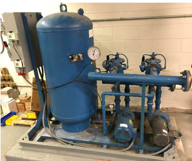
Cold Water Booster Pumps
