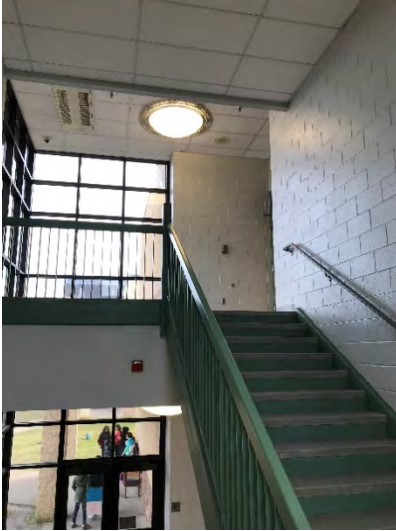
Staircase Decorative Lighting
