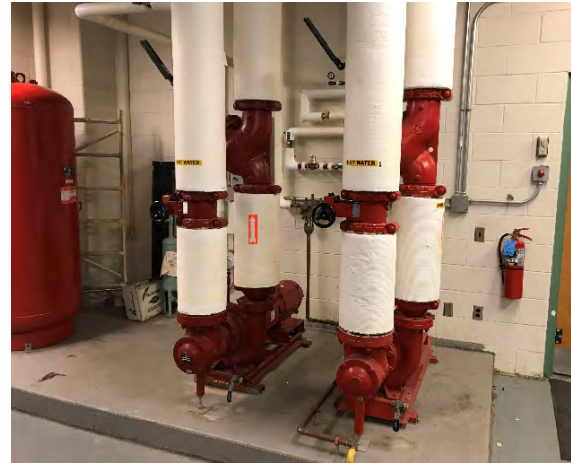
Heating Hot Water Pumps
