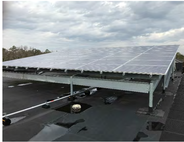
Solar Array on Roof
