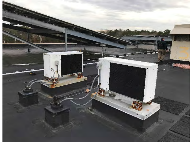
Condensing Unit for Split System
