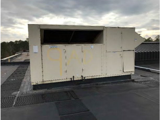
RTU on Roof
