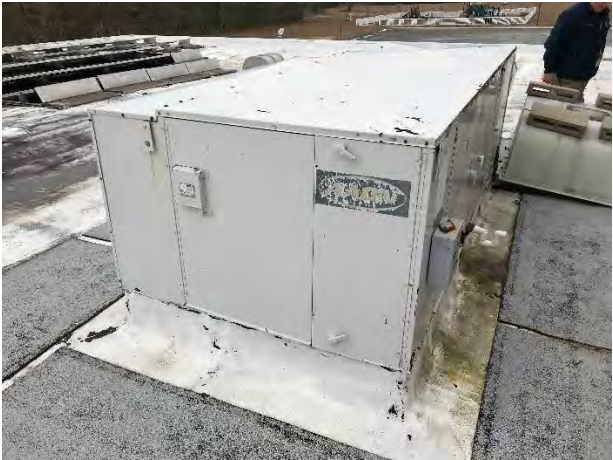
RTU on Roof
