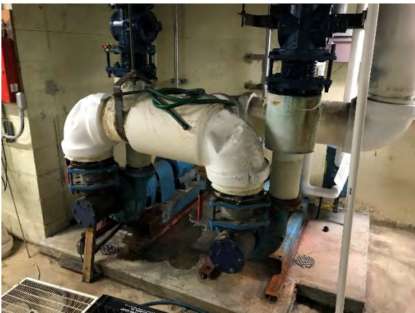
Heating Hot Water Pumps
