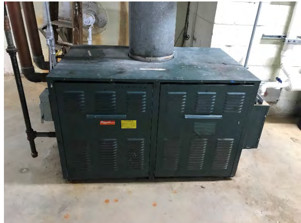
Hot Water Boiler
