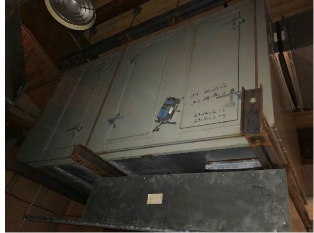
AHU in Gym
