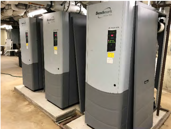
Condensing Hot Water Boilers
