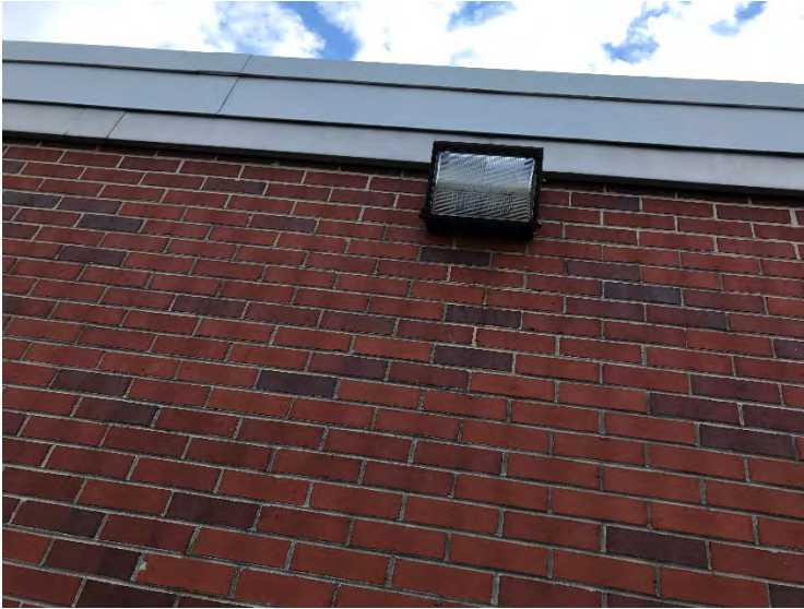
Wall-mounted LED Fixture
