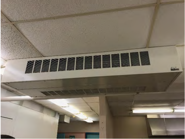
Fan Coil Unit in Kitchen
