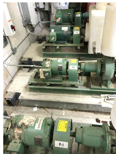
Heating Hot Water Pumps
