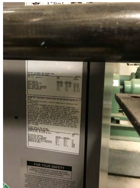
DHW Heater Nameplate
