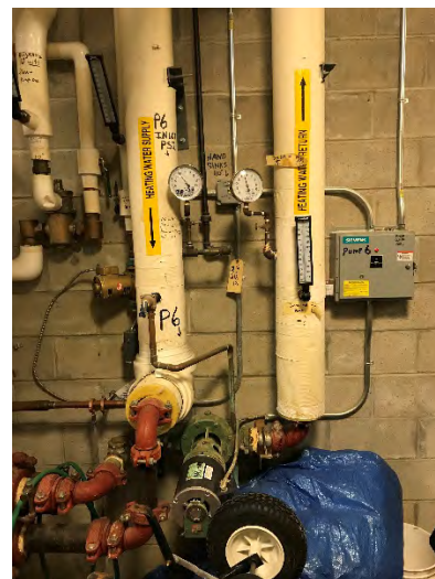
Water Supply Pump
