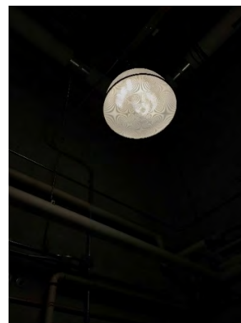
Boiler Room Lighting
