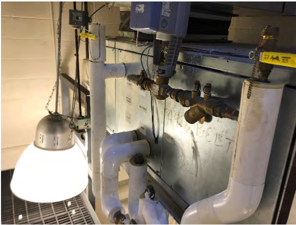
AHU-12 in Attic
