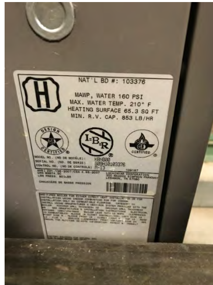
DHW Heater Nameplate
