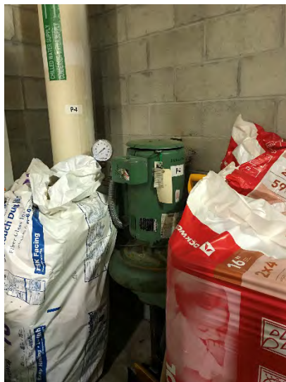
Chilled Water Pump
