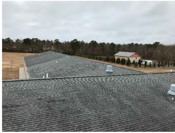
Shingles on Roof
