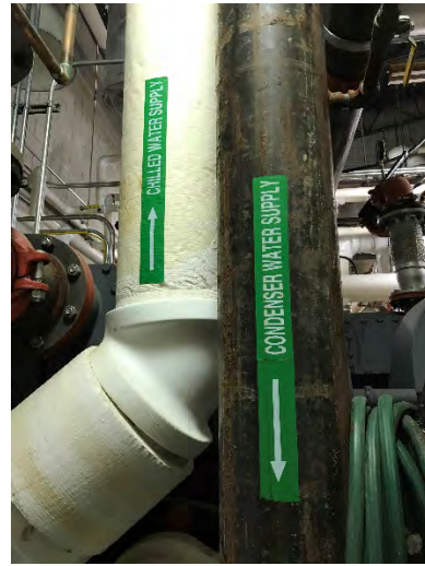
Chilled Water Pipes
