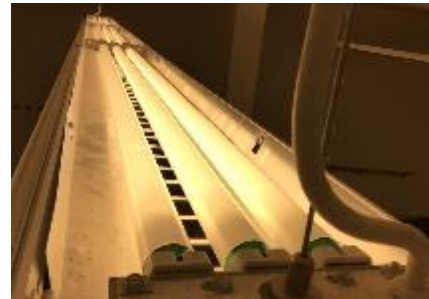
Linear T8 Tube Lights in a Hanging Fixture
