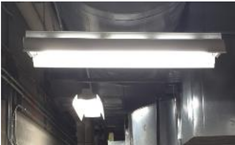
Hanging Fixture in a Mechanical Room
