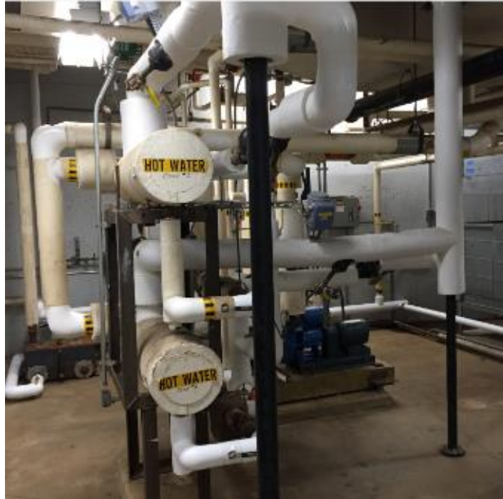
Hot Water Pumps & Piping
