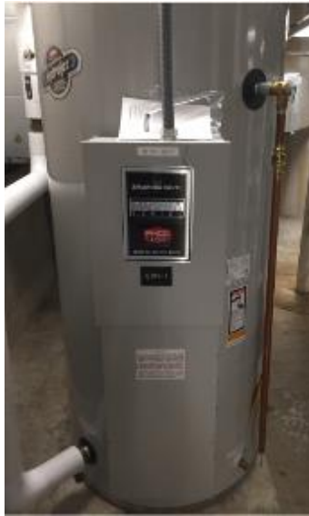
Electric Water Heater in Friends Center Basement
