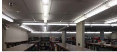
Linear Lighting Fixtures in Library
