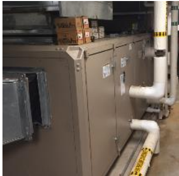
Picture of AHU-1
