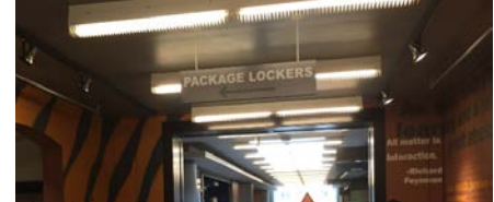
Interior Lighting Fixtures
