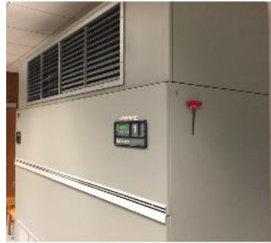
Picture of the CRAC Unit
