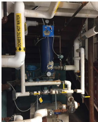
DHW Heat Exchanger
