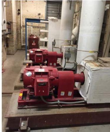
Chilled Water Pumps
