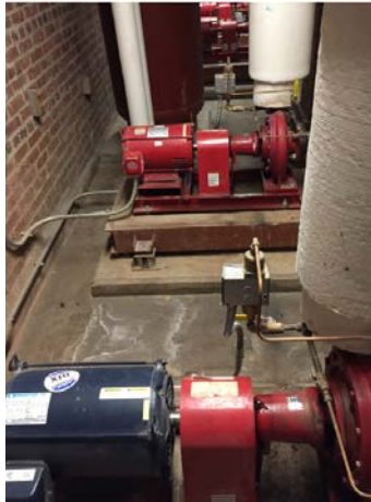
Hot Water Pumps
