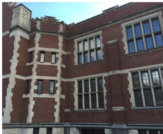
Exterior Walls & Windows
