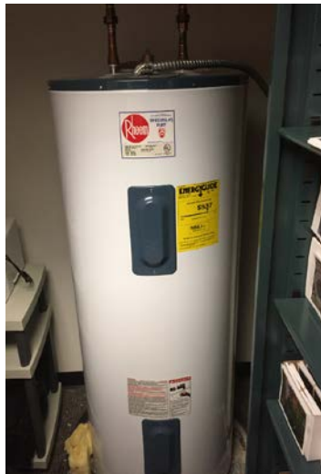
Electric Water Heater
