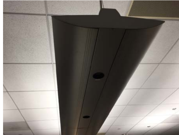
Indirect LED (tube) Lighting - Office
