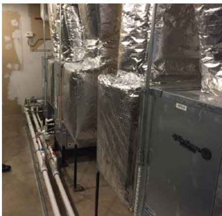
Water-Side Heat Pump (WSHP) Units
