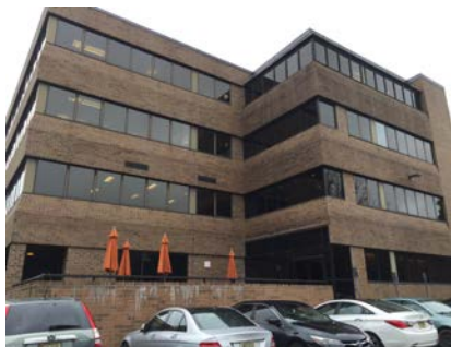
Building Façade and Windows
