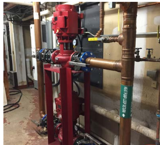
Heat Pump Water Loop Pumps
