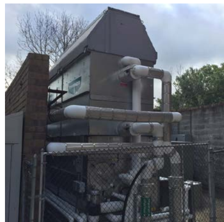
Cooling Tower (WSHP water loop)
