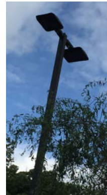
Pole LED fixtures
