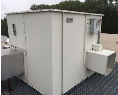
Make-Up Air Unit
