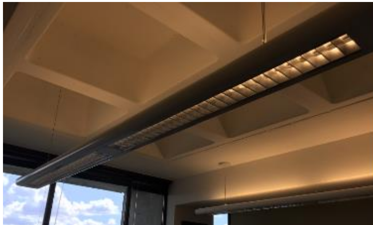
Suspended Fixtures with Linear LED Lamps
