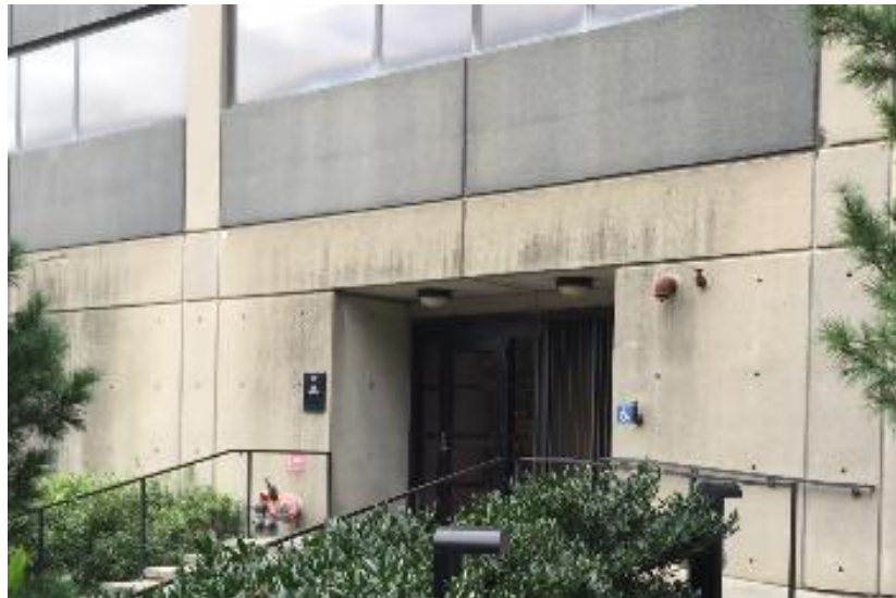
Picture of the Building Showing Exterior Walls, Doors & Windows
