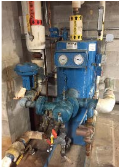
Steam to DHW Heat Exchanger
