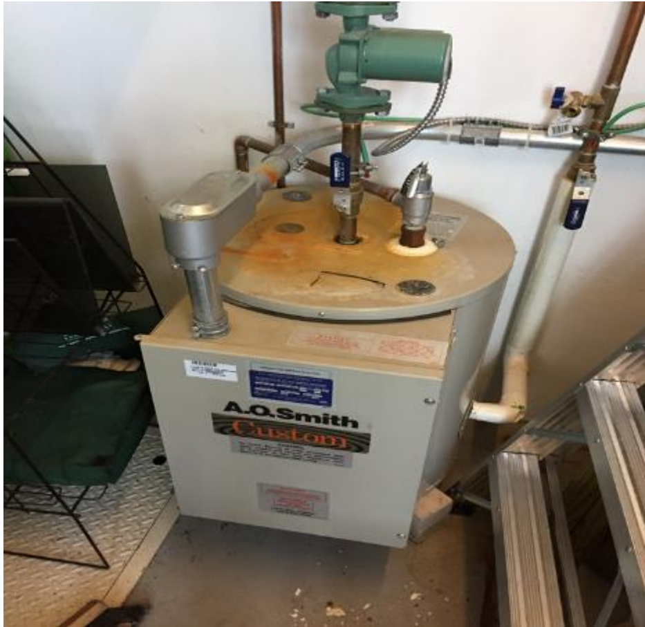
Image 3 Hot Water System
