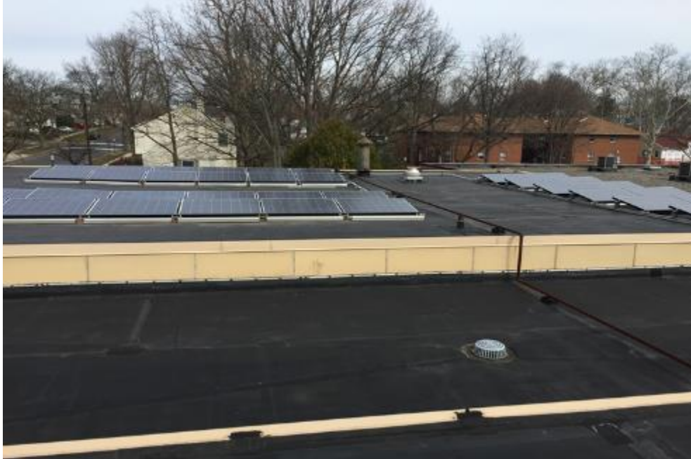
Image 3: Solar PV arrays
