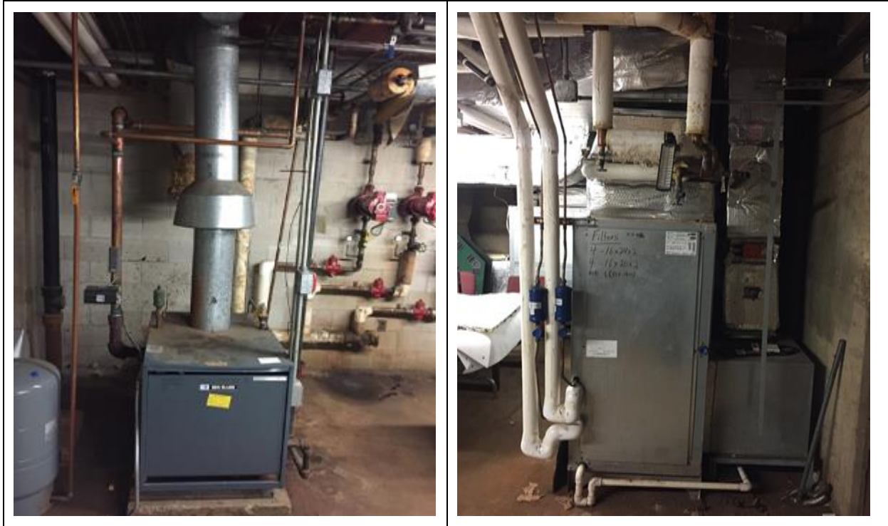
Image 5: Weil McLain Hot Water Boiler & Carrier Indoor Unit
