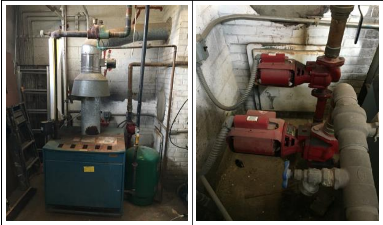
Image 4: Hot Water Heating System
