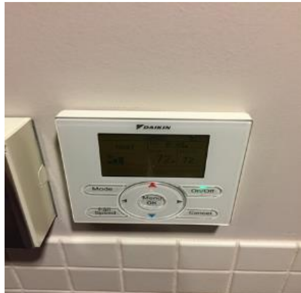
Image 6: Programmable Thermostat
