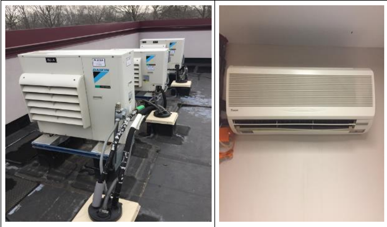
Image 5: Daikin Heat Pumps
