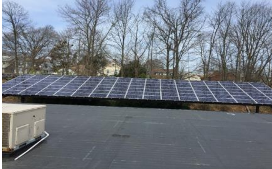
Image 2: Solar PV Arrays
