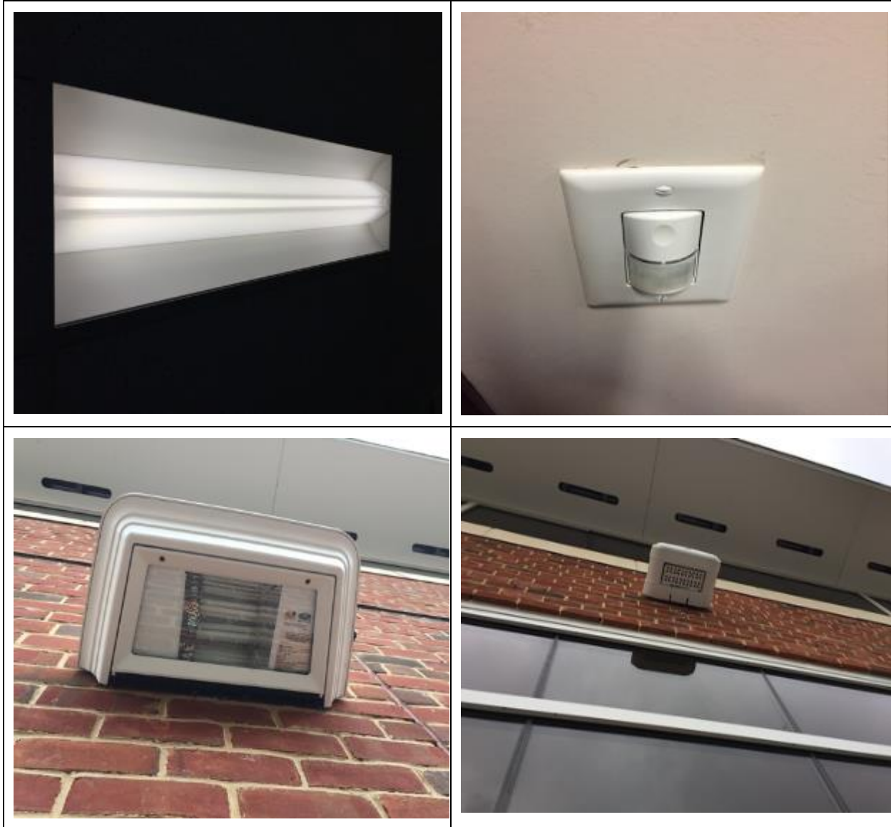
Image 3: Interior & Exterior Lighting System
