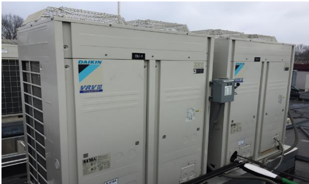
Image 4: Daikin VRF Heat Pumps
