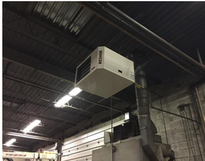
Image 4: Gas Fired Unit Heater
