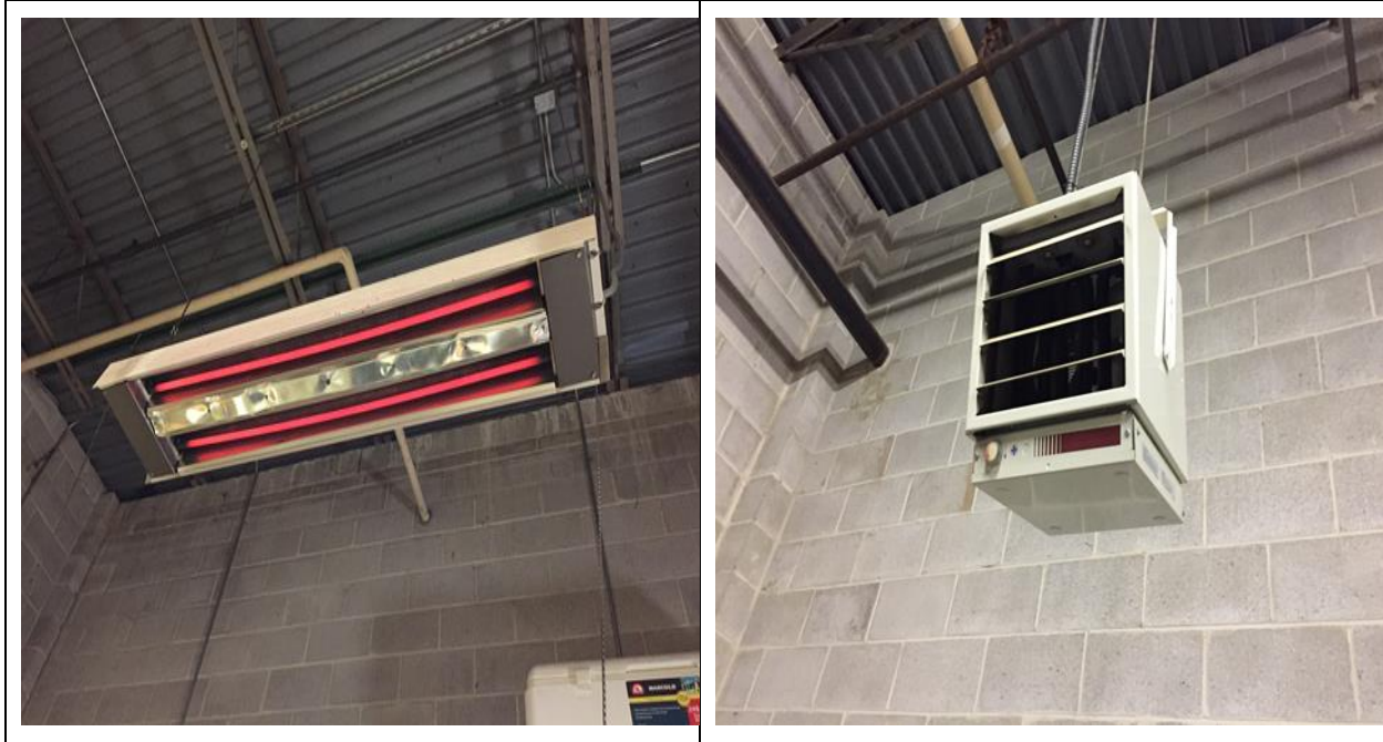
Image 3: Electric Resistance Heaters
