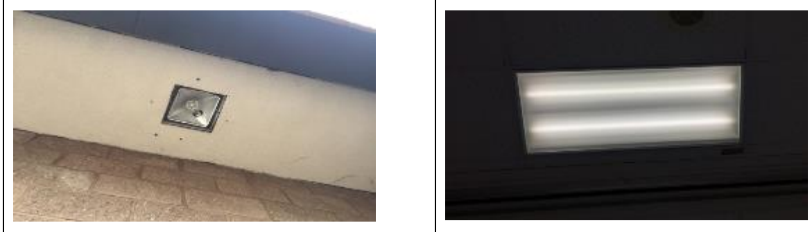
Image 2: Interior & Exterior Lighting System
