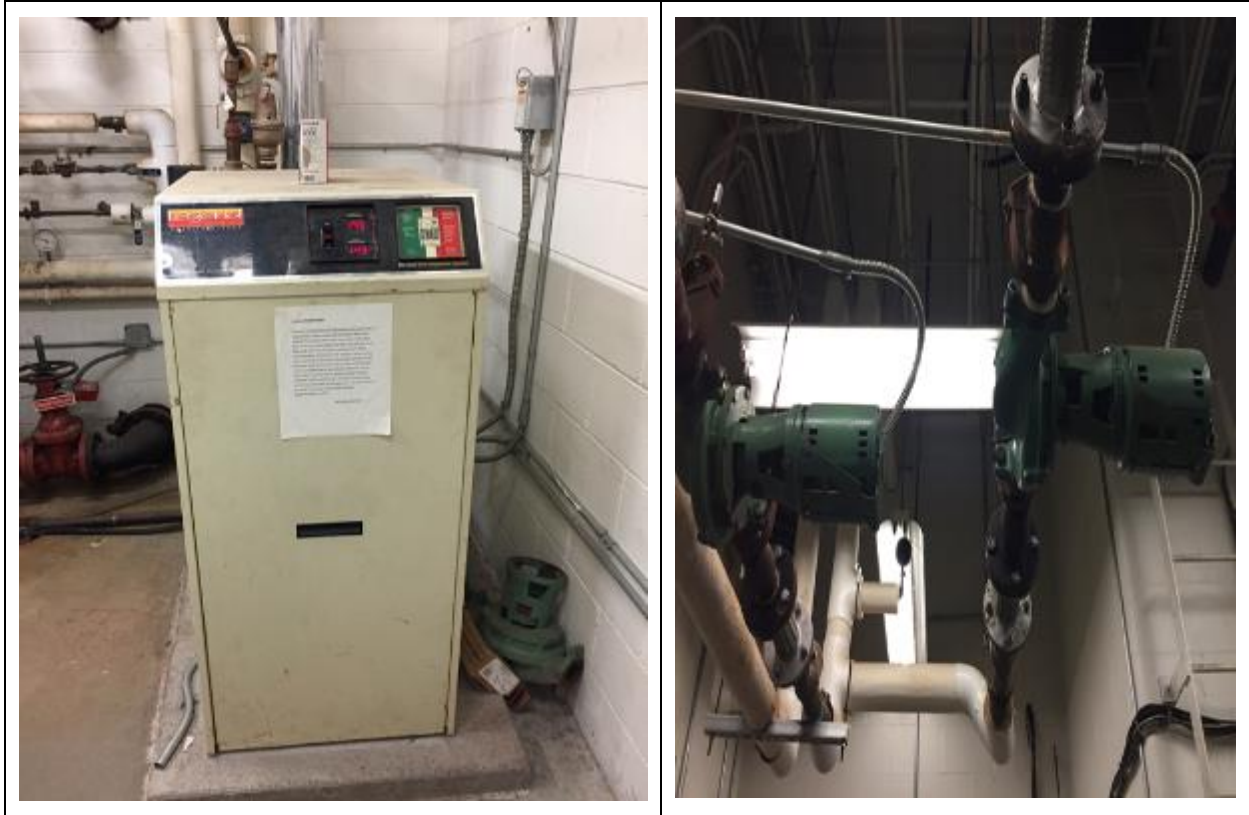
Image 3: Hot Water Heating System
