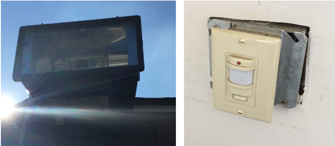
Image 3: Exterior metal Halide Fixture & Occupancy sensor
