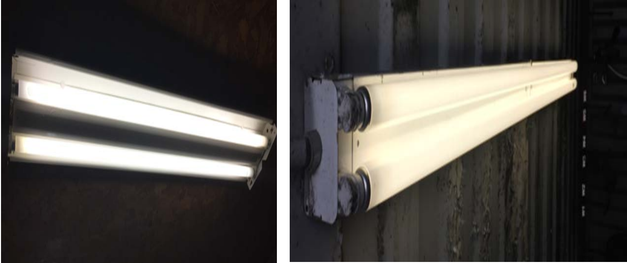
Image 2: Interior T8 and T12 lamps
