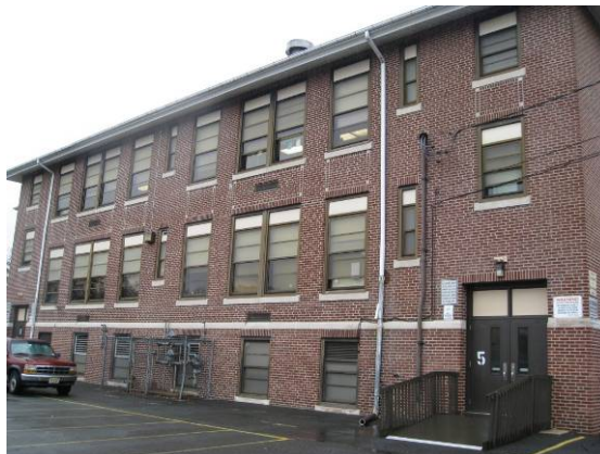
Brick exterior on back of school
