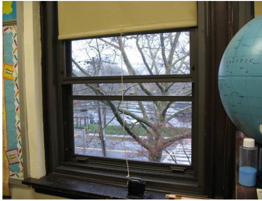
Typical classroom window
