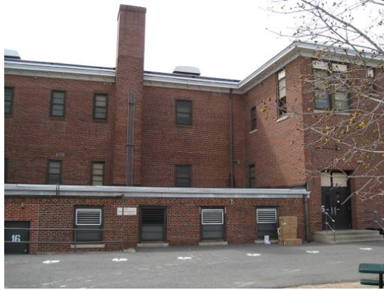
Various wall penetrations
