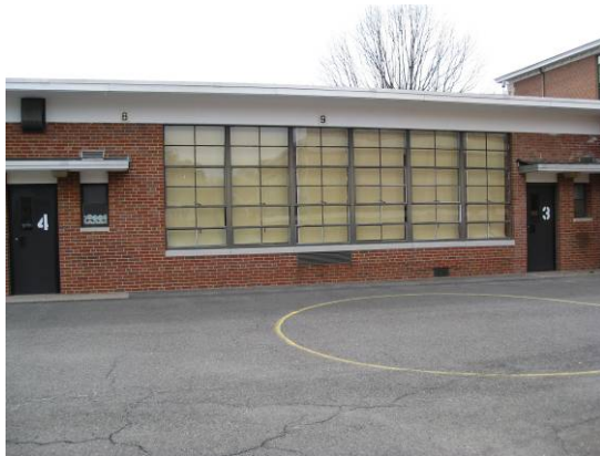
Old Steel Frame Single Pane Windows
