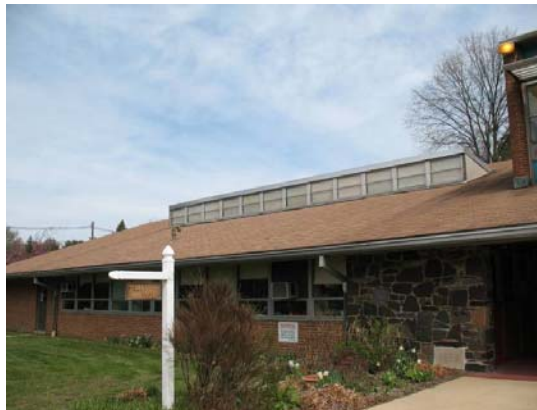
Asphalt shingle roof
