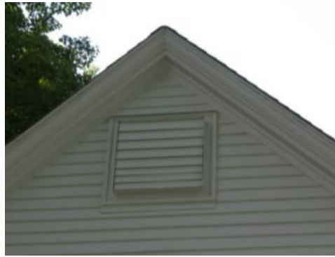
Gable End Louvered Vent were found to be either partially clogged or closed at the time of the field visit
