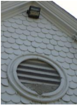
Gable End Louvered Vent were found to be either partially clogged or closed at the time of the field visit
