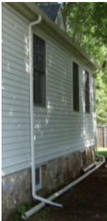
Gutter Extension should be directed away from Exterior Walls
