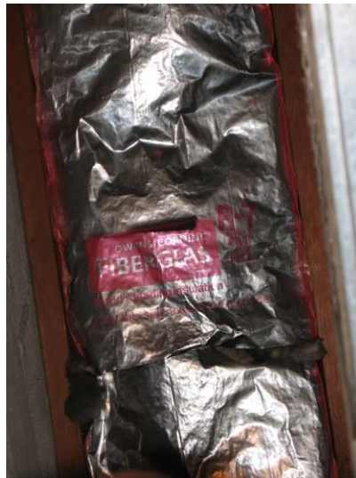
Foil faced fiberglass insulation 2 ¼ inch R-7 in roof rafters
