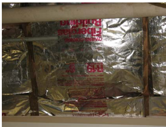
6” Foil-faced fiberglass found in rafters in 2 nd Floor Mechanical Room
