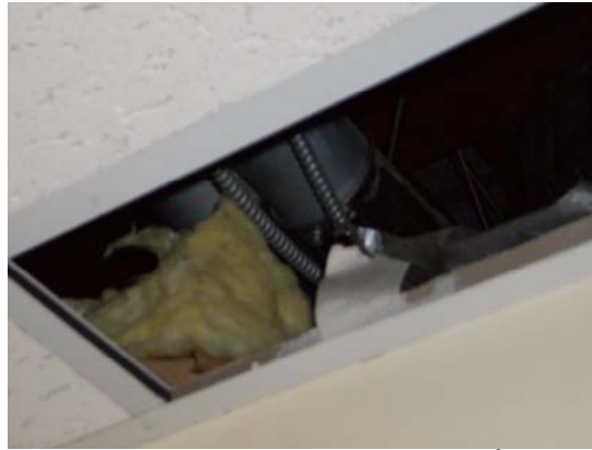
Fiberglass above ceiling tiles on 2 nd floor
