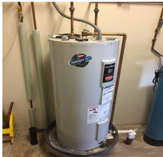
Image 5: Domestic Hot Water Heater
