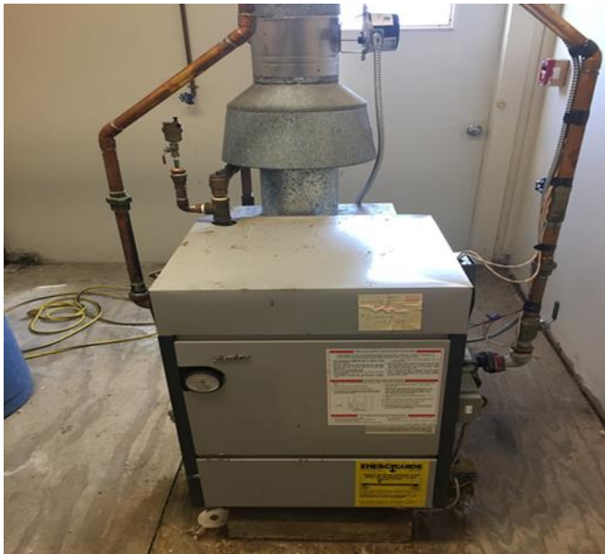
Image 3: Propane Fired Hot Water Boiler
